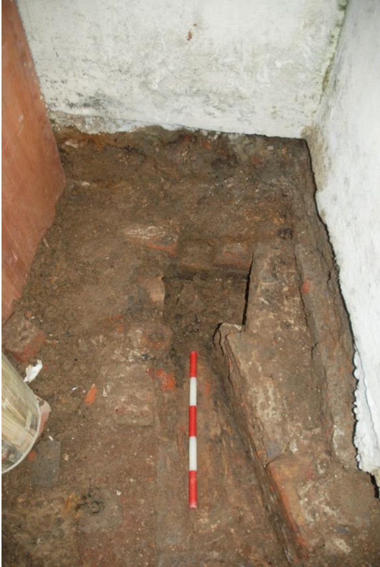
Figure 8: Square part of the drain, filled by silty soil. Facing E. Scale 0.5m.
