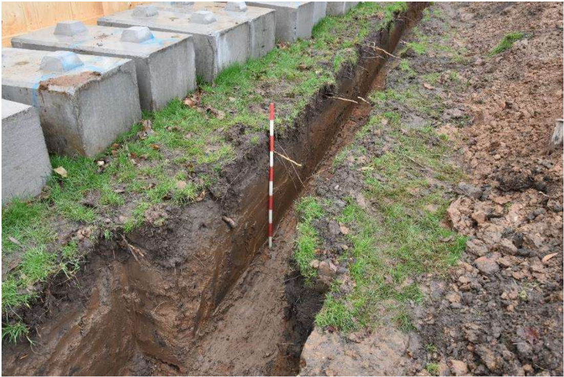
Figure 26: Section of service ducting along the southern perimeter (Trench 13) showing topsoil (1) and subsoil (2) over natural clay (57). Facing SW. Scale 1m.
