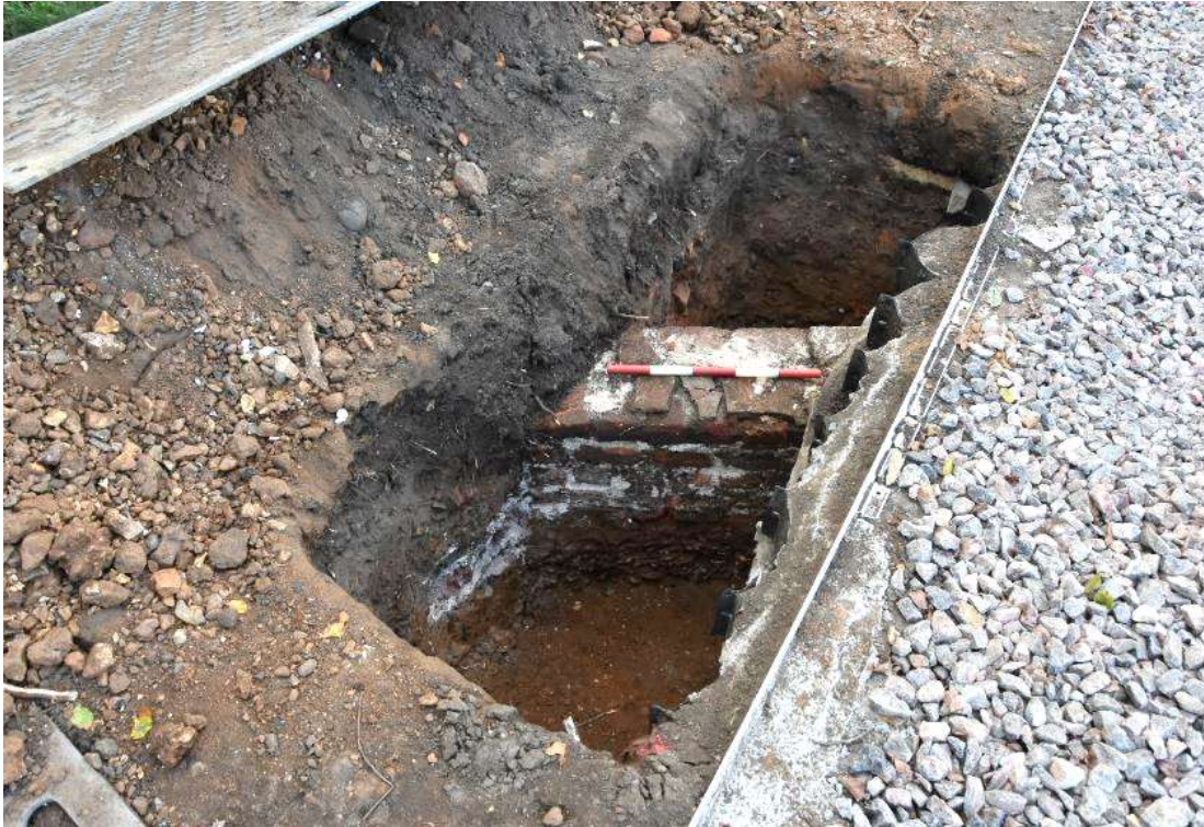
Figure 18: Slightly neater north-east face of wall [17]. The messy patch of mortar may indicate a partial rebuild. The tile course can be seen beneath the scale. Facing SW. Scale 0.5m.
