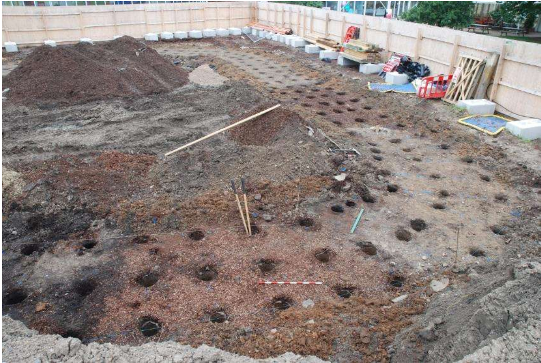
Figure 31: Completed post holes undertaken prior to the erection of the Boardwalk, located in the northeast corner of the site. Facing NE. Scale 1m.
