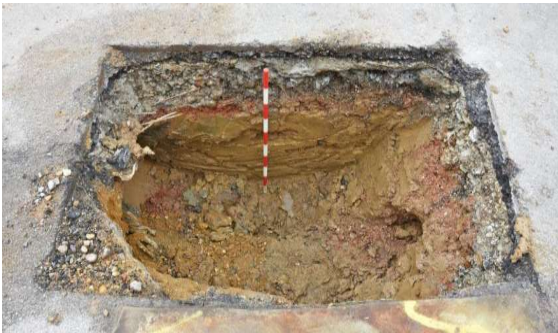
Figure 7: The same stratigraphy was encountered towards the southern end of Lyncroft Gardens, comprising the existing road surface above reinforced concrete and rubble, overlying the natural geology. Facing NW. Scale 1m.
