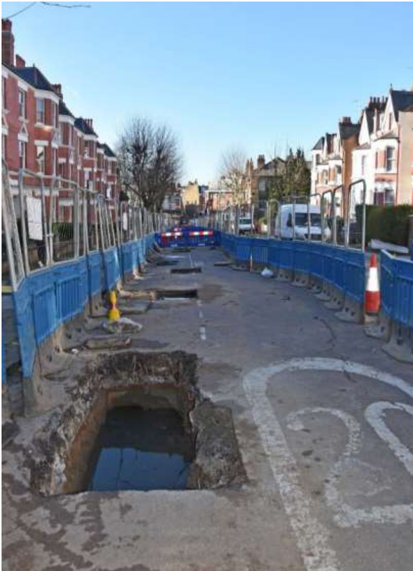
Figure 5: Completed pits, looking towards Fortune Green Road. Facing SSW. No scale.
