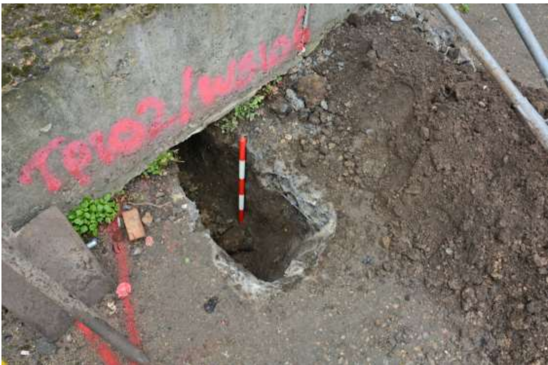
Figure 10: TP102, showing made ground below concrete. Facing NW. Scale 0.5m.
