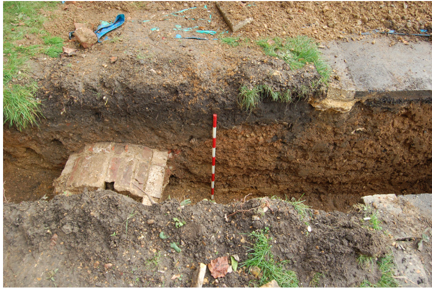
Figure 23: Trench 7 looking west. Arched brick drain [3] within linear cut, truncating redeposited gravel backfill (1m scale).
