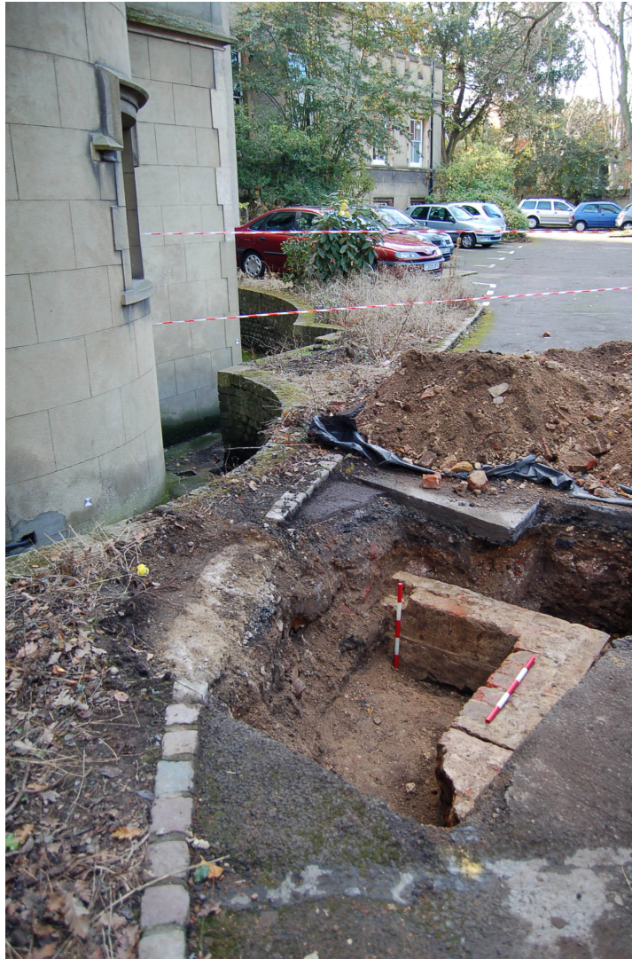
Figure 36: Trench 9, view south-west – showing relationship of walls [4] and [5] with existing building.
