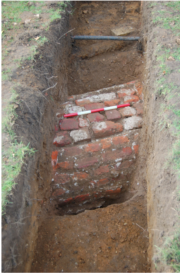
Figure 18: Brick built drain in Trench 3, view looking west (0.5m scale)
