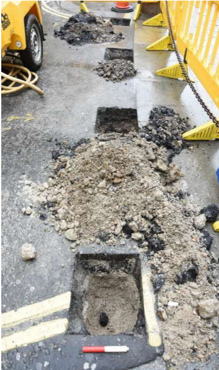
Figure 15: Completed trenches. Facing W. Scale 0.2m.
