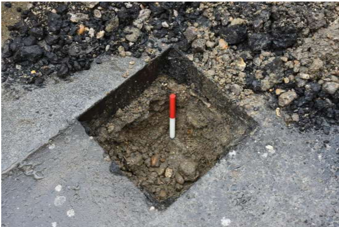
Figure 17: Completed trench. Facing NE. Scale 0.2m.
