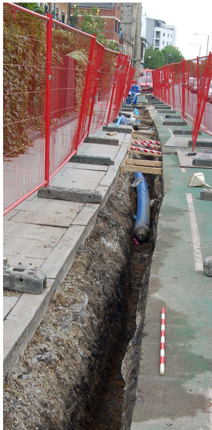
Fig. 7 Trenching in Cable Street, looking west
