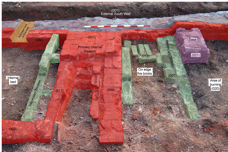
Fig 23 Detail of central deposits in Bay 7, showing in red the more major structures adjacent to main wall foundation [001] (at the top of the picture with the scale lying on
