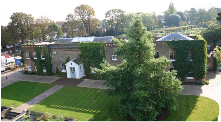
Fig 16 The Georgian Grade II Listed former fruit store building, view looking southeast. Restoration works in the 1960s replastered much of the brickwork (much in cement) and the original flush pointing style (possibly ‘penny point’) cannot be seen. © John Lonsdale, RBG Kew.
