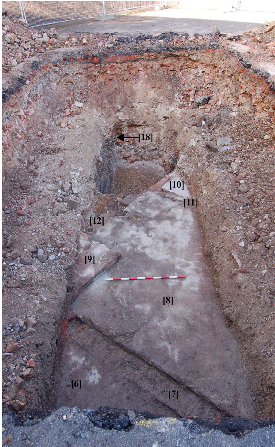
Figure 8: Trench 1, view north showing the series of walls and concrete slabs. (Scale 1m)
