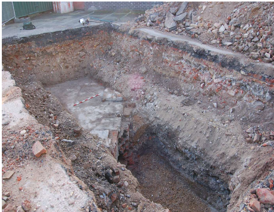
Figure 11: Section and view of Trench 1.
