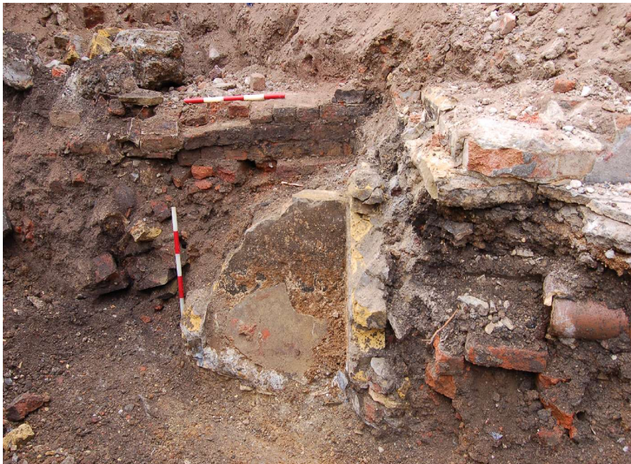
Figure 13: Trench 1 view southwest showing drain chamber [25], ceramic drain [27] and deposit [24] below concrete slab [8] and wall [7].
