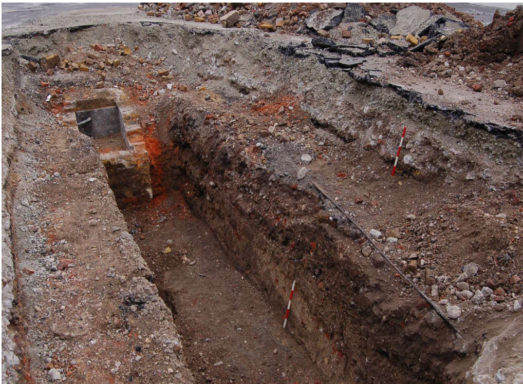
Figure 14: Trench 2 view east.
