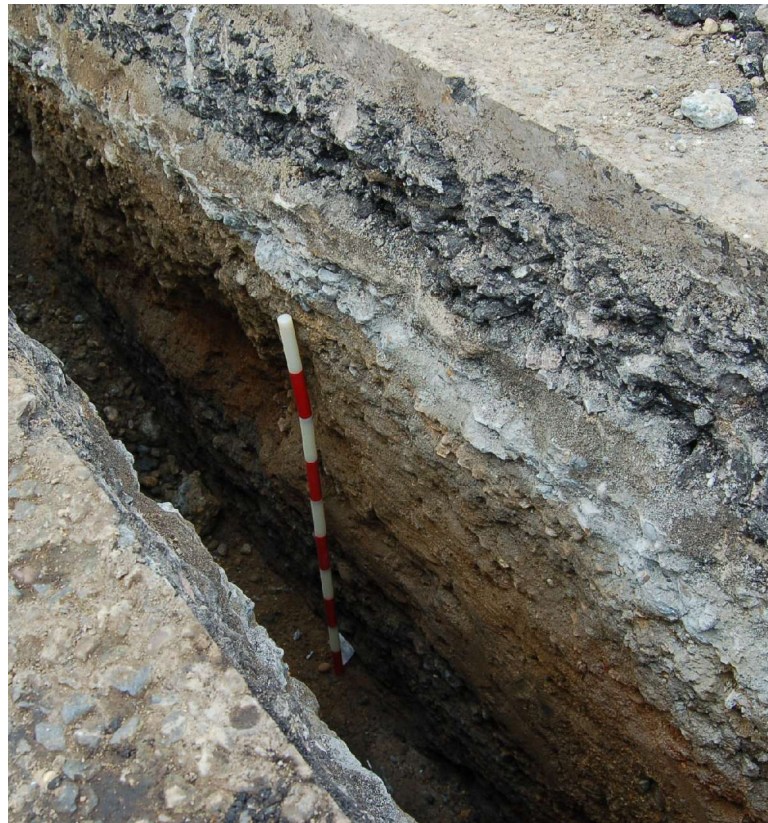
Figure 4: Southeast facing section of the southwest end of Trench 1. Showing tarmac and base [1] overlying hardcore [2], and made-ground layers [3] and [5].
