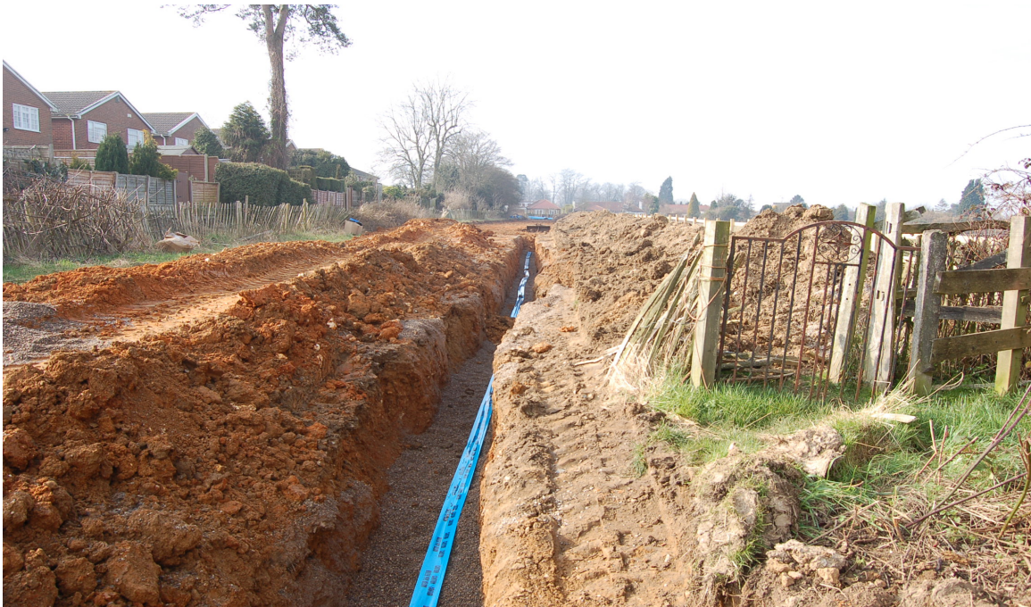
Fig 6. The watermain lying within its trench at the junction between the Access Road and the easement track.
