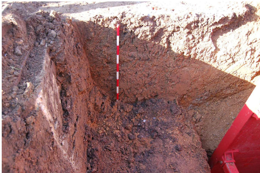
Figure 7: East facing section of open cut pipe trench.
