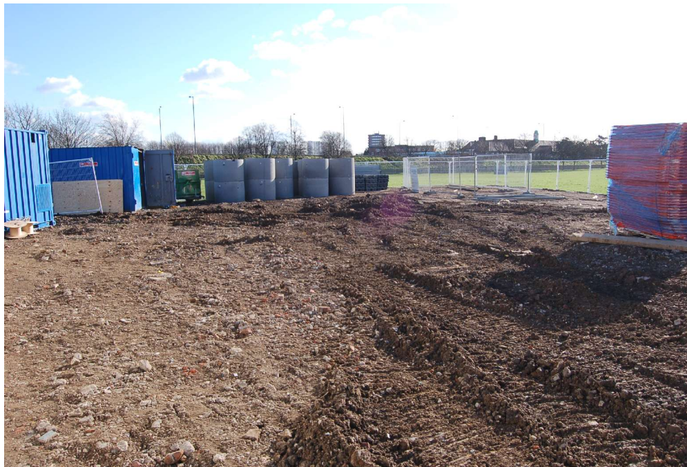
Figure 3: The site compound area.
