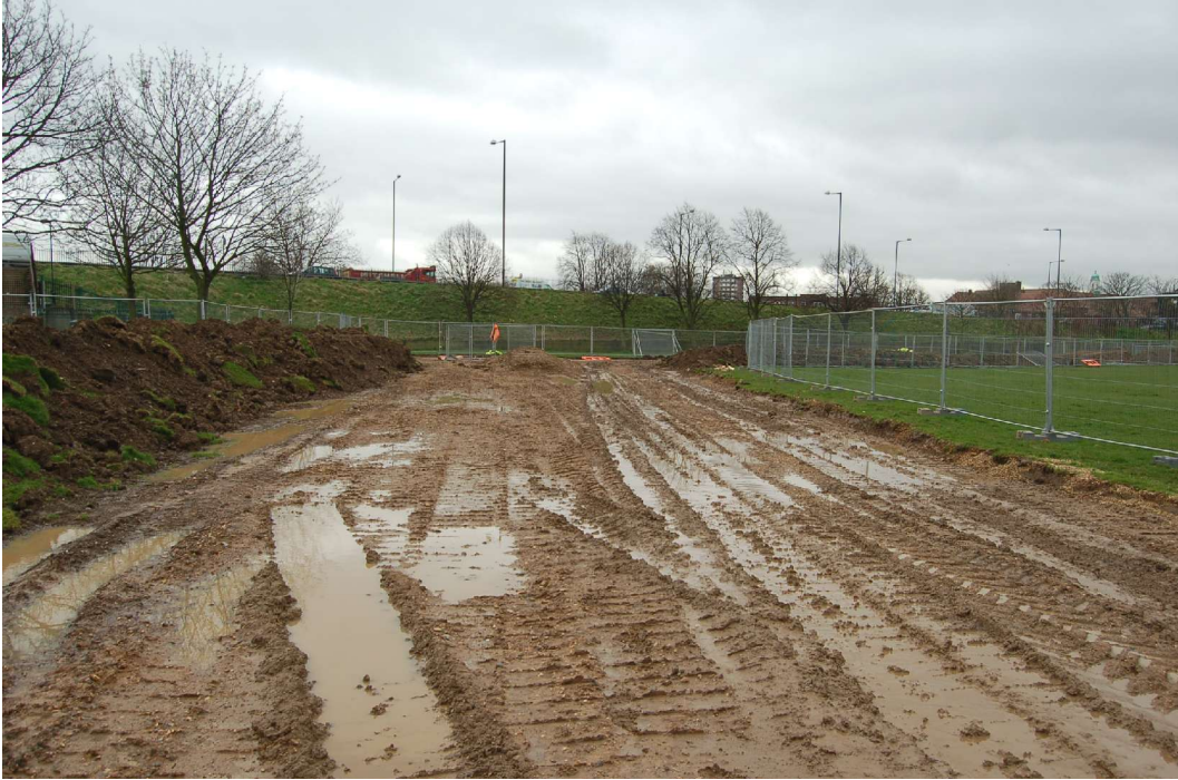
Figure 5: Stripped ground in the south of Area 2, view looking southeast.
