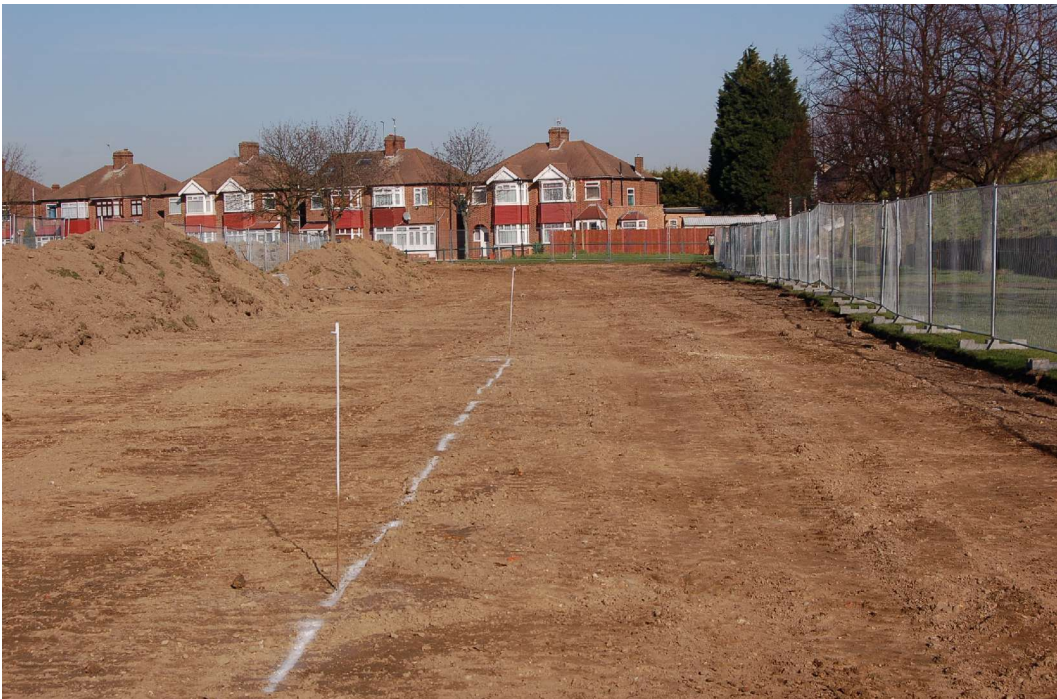
Figure 6: Stripped ground in the south of Area 2, looking northeast.
