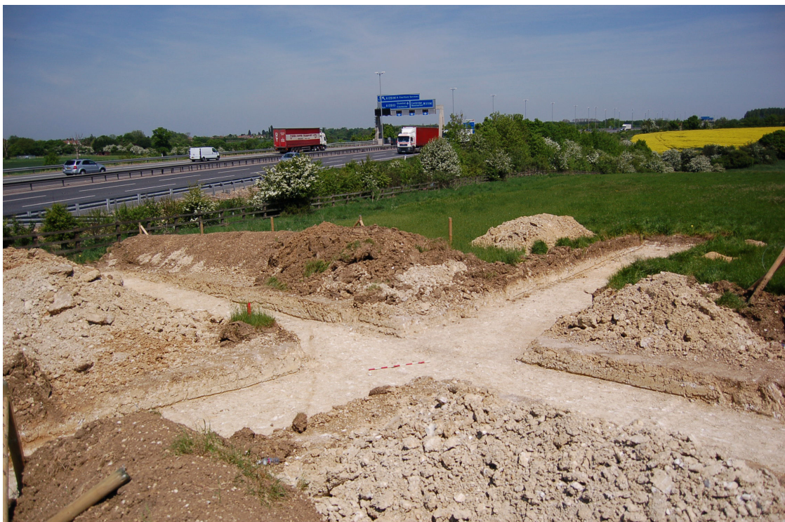
Figure 18: Overall view of Trench 1, looking north-west towards the M11.
