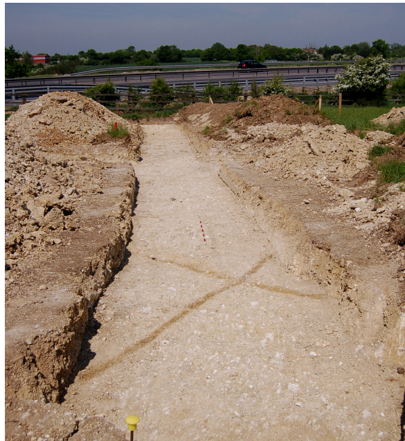
Figure 8: View west towards the M11 of Trench 1, showing plough furrow [20] and linear feature [22] (1m scale).
