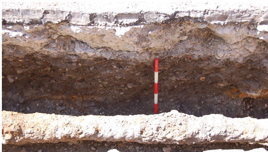
Fig.10 East-facing section outside No. 212 Deptford High Street, with a corroded cast iron pipe exposed in the foreground. A further iron pipe is visible in section either side of the 0.5m scale
