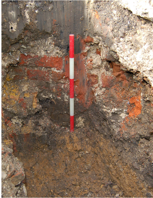
Fig. 9 The east facing section of test pit 8 showing the in situ brickwork (scale: 0.5m)
