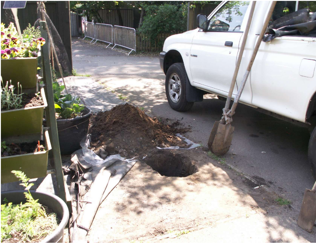
Figure 6 Detail of the area of Test Pit 2.
