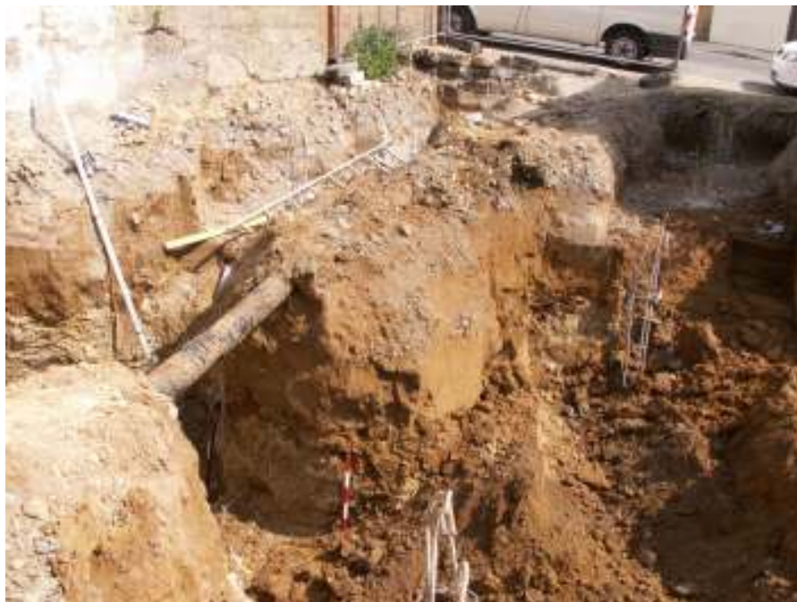
Figure 17 The groundworks in the northern corner of the site, looking north
