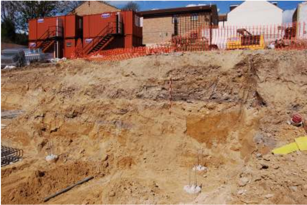
Figure 16 The south facing section crossing the site, the bank separating the northern higher terrace from the lower level, is visible in the foreground. Recent made ground deposits can be seen directly overlying truncated natural sands.
