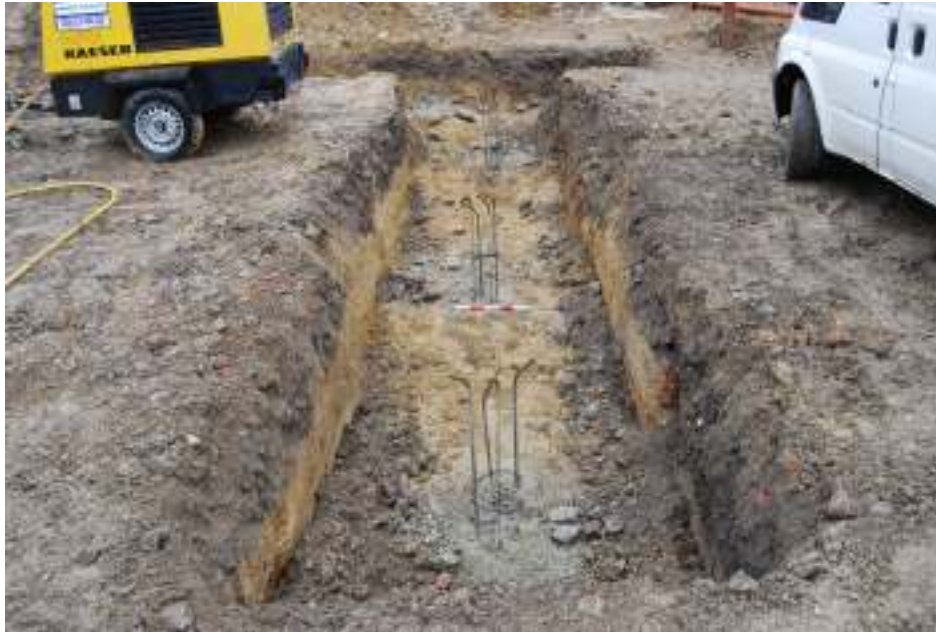
Figure 13 Trench 5, looking northeast
