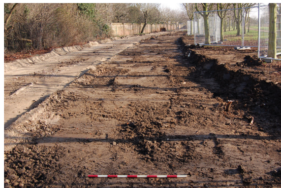
Fig 5: General view looking southeast of the 'horse ride' after the completion of the preliminary topsoil stripping.
