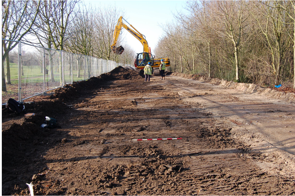
Fig 4: General view looking northwest from the area of manhole No.10.
