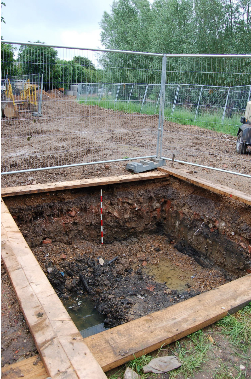
Fig 10: View of manhole No.5 looking south.
