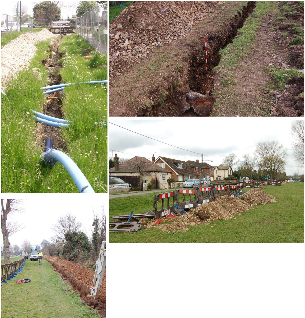
Fig. 8 General views of trenching works in the Green Street Green area:
