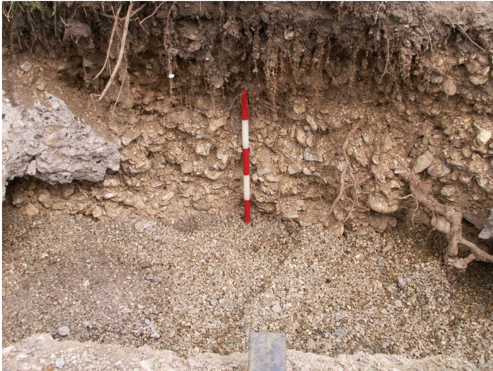
Fig. 12 Localised trenching on the north side of Green Street Green Road and just west of the junction with Canada Park Road ( 0.5m scale )
