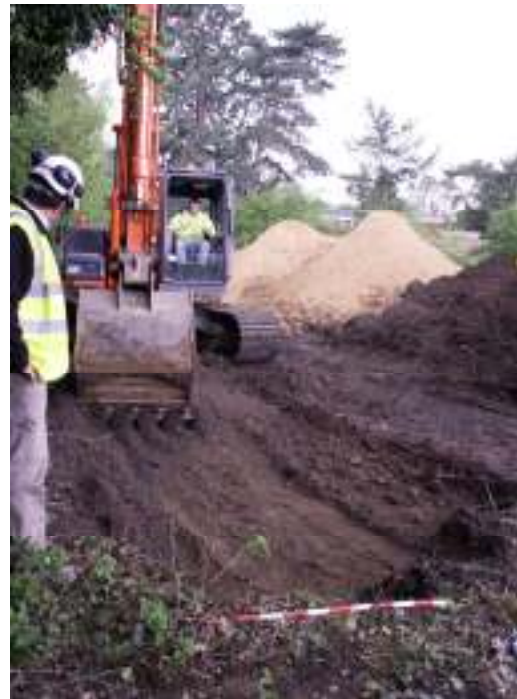
Fig 7: View looking west of the topsoil stripping in the area west of manhole BPSW7.
