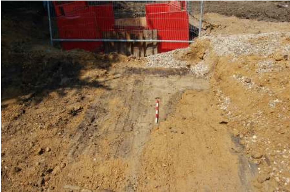
Fig 8: View looking west towards manhole BPSW7, showing the clay and natural sand that was visible at a depth of 550mm.
