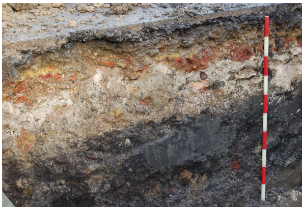
Fig 6: An oblique view of the south-facing section showing the possible earlier road surface beneath the tarmac and the underlying silty alluvial deposit.
