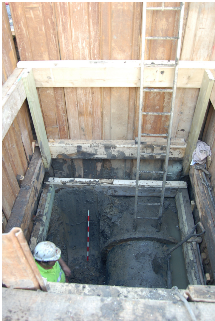
Fig 9: A post-excavation picture showing the exposed 42'' trunk main ( 1m scale ).
