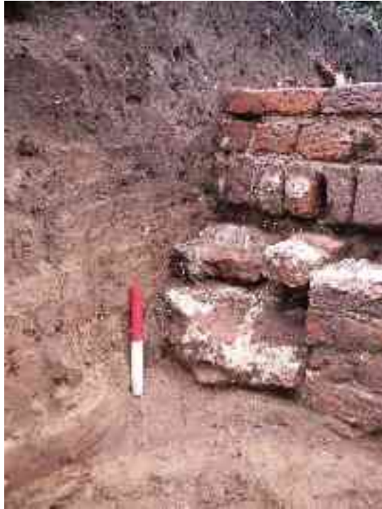
Fig.21 The construction cut/s [21& 22] in the east facing section at the northern end of Trench 6. Note also the differently oriented pad base at the trench edge relative to the others in previous photos and the gravel adhering to the top of the pad base to the right of the image (scale: 0.2m).
