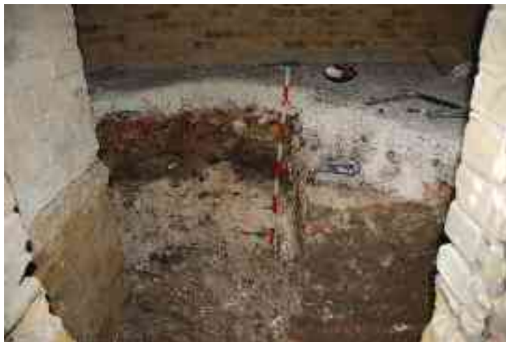
Figure 69: Section in the extension cubbyhole showing concrete and made-ground layers.
