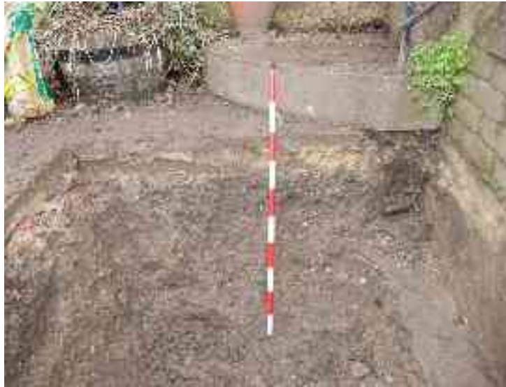
Figure 68: South facing section showing concrete slabs over bedding with made-ground deposits beneath (1m scale).
