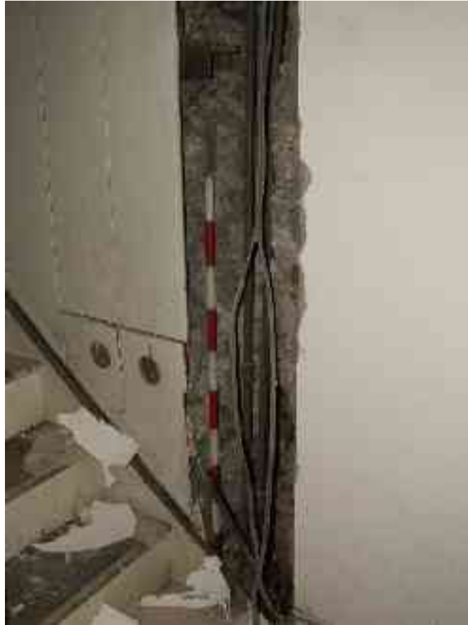
Figure 31: Exposed brickwork at the bottom of the staircase on the lower ground floor.
