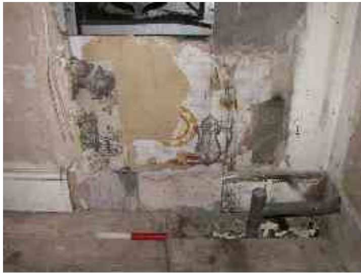
Figure 38: Missing plaster and skirting in the corner of the kitchen extension.
