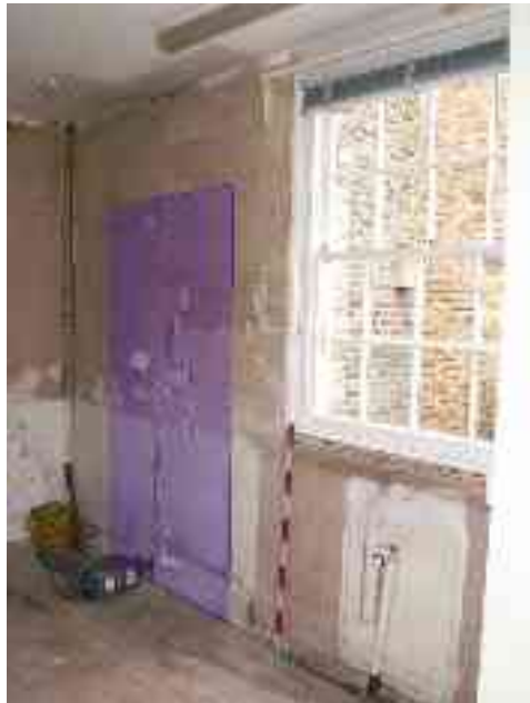
Figure 37: Existing window to be blocked up and location of new glass doors onto raised patio.
