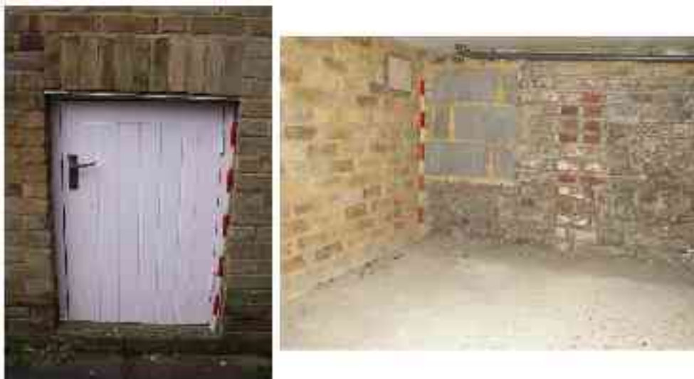
Figure 17: Cubbyhole storage space below the 1970s extension, inside showing blocked-up window in the earlier Victorian brickwork.
