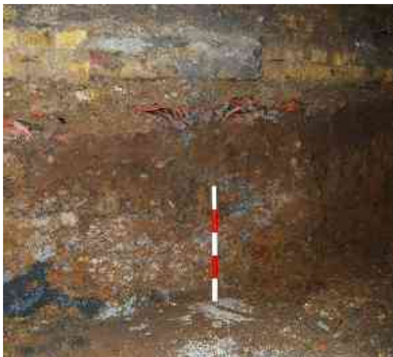
Figure 19: Section One showing the existing wall and associated foundation layers overlying truncated natural sand and gravels ( 0.5m scale ).
