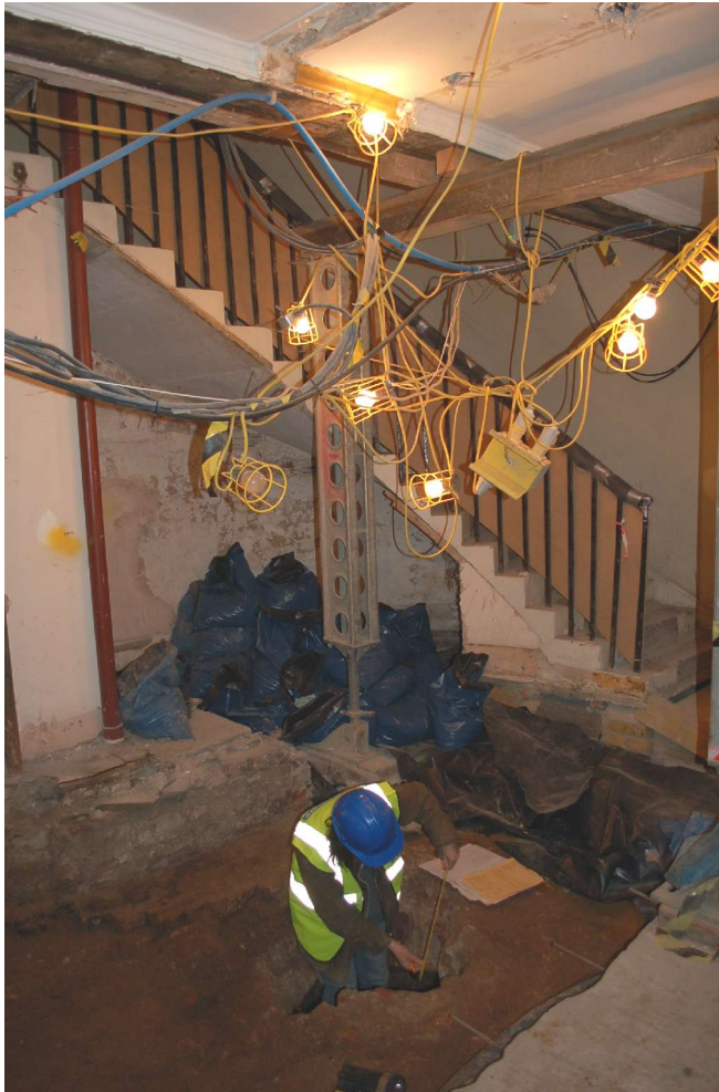
Fig 14 An archaeologist records the roughly circular domed cistern. Note the location, just below the existing basement floor and just to the south and east of the main staircase access to the basement. The figure is standing inside the feature where a main timber upright support to the overlying floor previously stood. The timber upright was slightly off centre with the crown of the cistern. The cistern measured an approximate internal diameter of 1.36m (just over 4ft) and was initially recorded to a total depth of 1.7m (5ft 7" cf. Fig 13). In profile the sides of the cistern were not completely vertical, but at the neck - between the shaft of the well and the overlying crown - the walls tapered slightly so that the profile increased by about 150mm towards the crown, in this location the internal diameter of the well was 1.40m, beyond this depth the walls were broadly vertical. This slight expansion in diameter may have perhaps helped to hold the former or falsework for the domed crown above or was simply to make the top of the well slightly wider. A similar circular cistern of 19 th century date and 4ft diameter has been recorded as having the capacity to store between 78 and 98 gallons of water 27 . The cistern was constructed of red stock moulded bricks (mainly seconds) and was dry lined, but with a mortared domed crown partially surviving.
