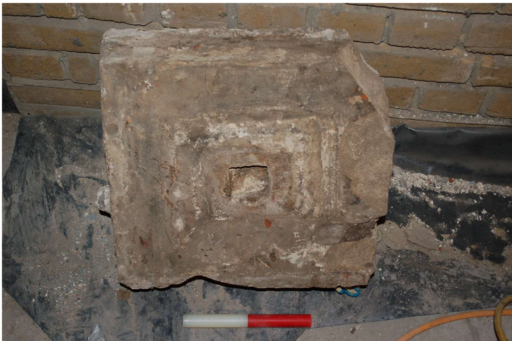
Fig 18 The rectangular Oolitic limestone block discovered on top of the domed cistern. The visible face is the upper face and the base of the block is roughly hewn.
