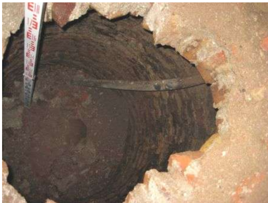
Fig 13 The original discovery of the cistern in early February 2009, showing the lead pipe and the original depth of the feature c 1.7m. The feature was partially backfilled for health and safety reasons. © Stephen Gray, Weldon Walshe Architects.
