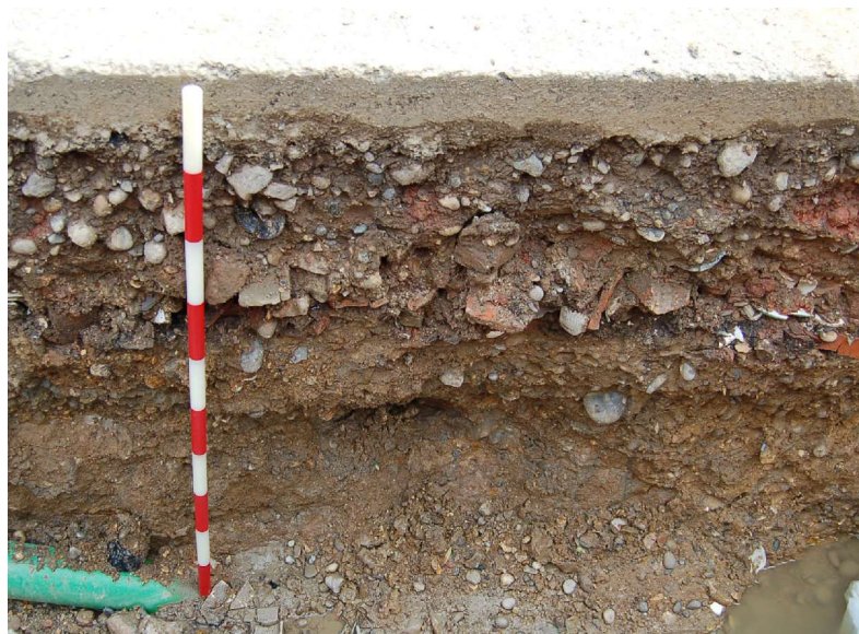
Figure 8: Section of trenching on West End Lane (04-10-08) showing rubble road makeup containing 19 th century building materials and pottery.
