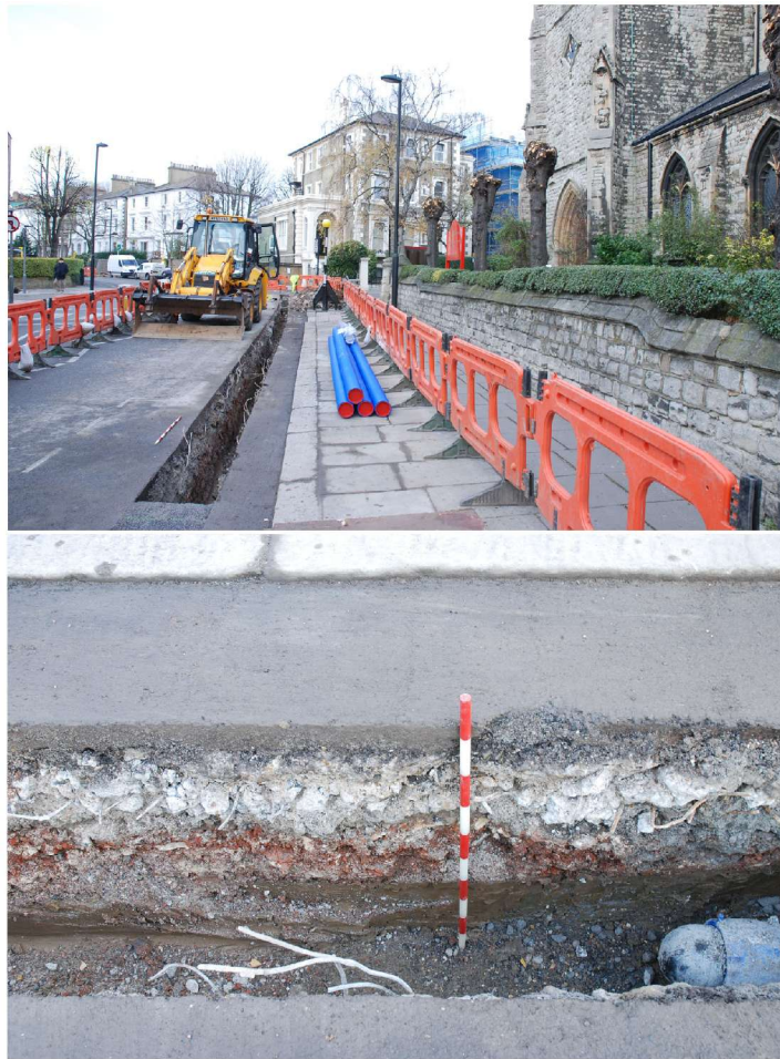
Figure 20: Trenching on Abbey Road.
