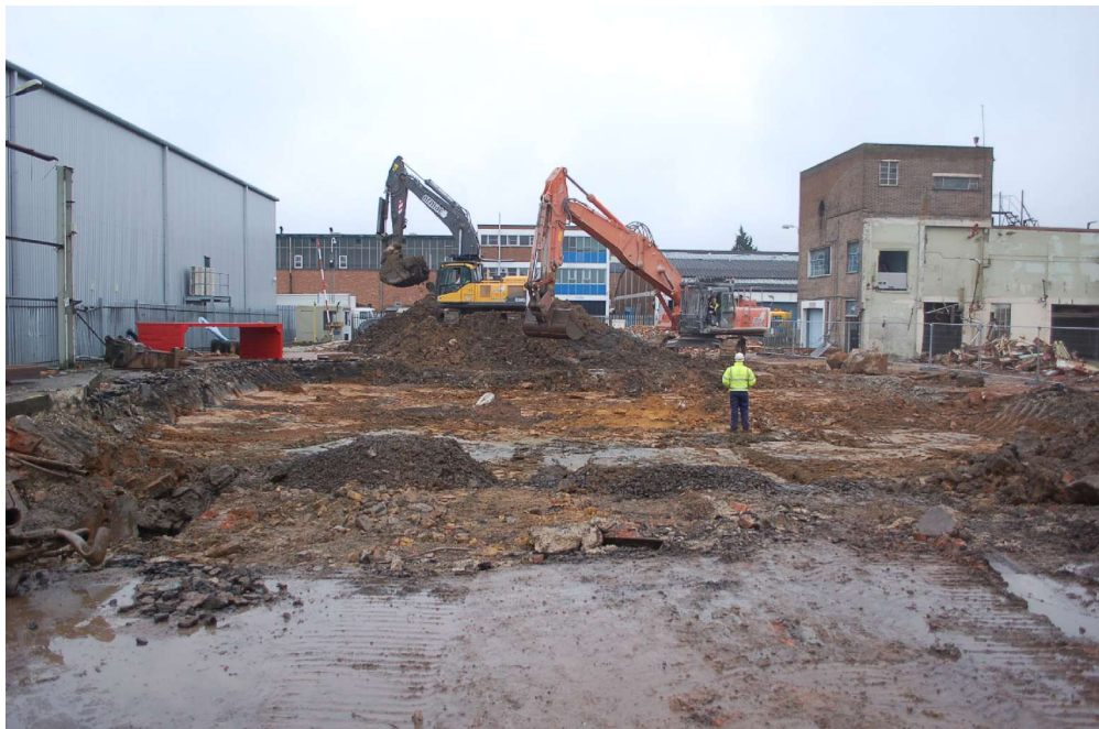
Figure 21: View south towards Progress Way of Open Area Trench WS3
