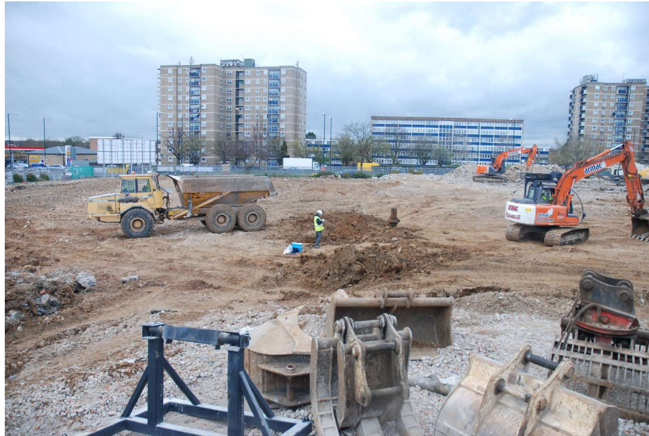
Figure 16: View looking west of Quadrant C towards Great Cambridge Road.
