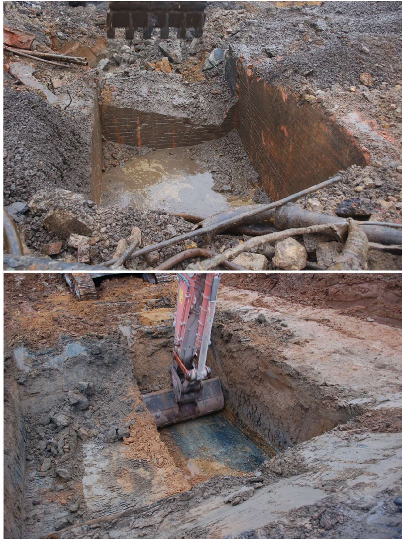
Figure 22: View of WS3, water-filled modern brick chamber (top) and smaller excavated area prior to trench boxing showing natural gravels (bottom)
