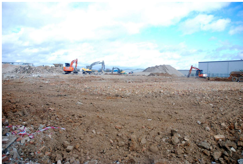
Figure 9: View looking northeast of Quadrant B.
