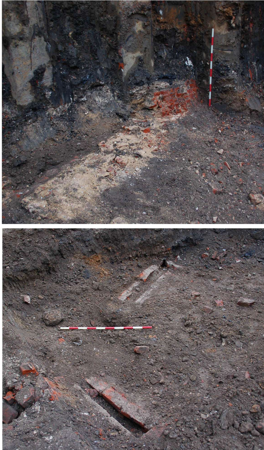
Figure 11: Victorian features observed during initial machine reduction; brick foundation (top) and brick drains (bottom).
