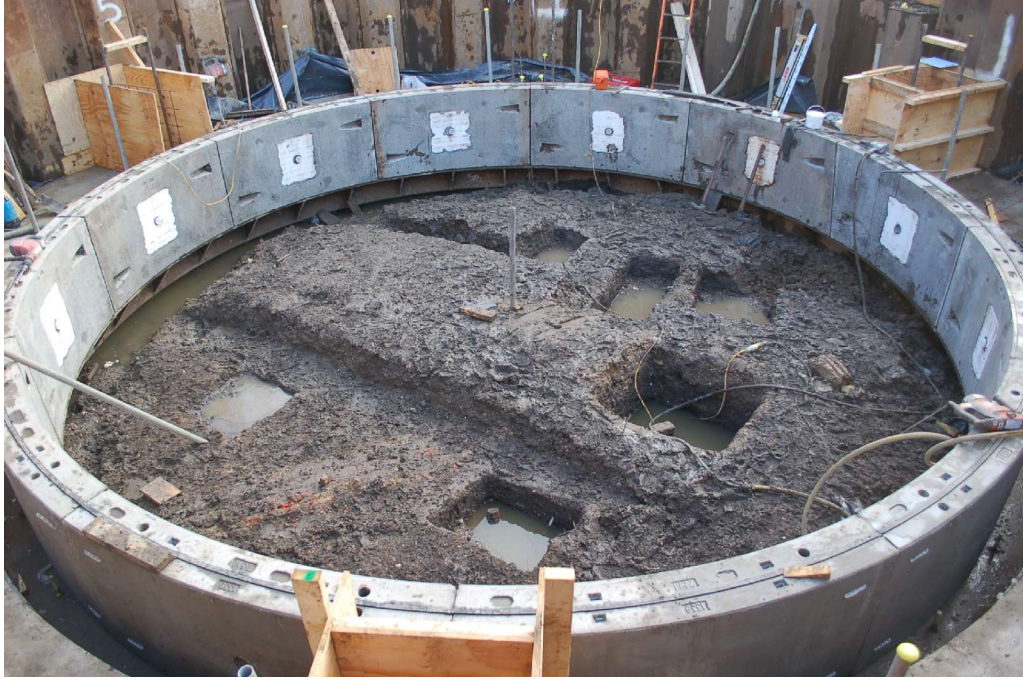
Figure 15: Looking south east with Test Pits 3 and 2 in the foreground.
