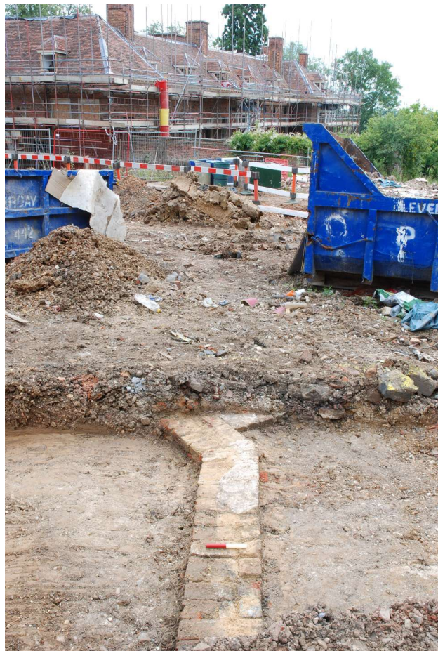
Fig. 19: Trench 3, view looking east along the line of wall [15] ( scale 0.2m )
