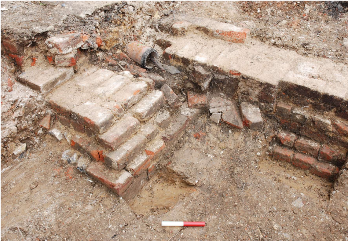
Fig. 28: Trench 4. Detail of the northwest end of the exposed wall base [10] (scale 0.2m)
