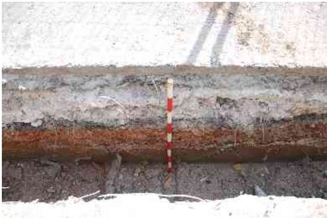
Fig 9: A north facing section of the mains replacement works showing a thick red made ground deposit below the road surface in Ladbrooke Grove ( 1m scale ). The truncated surface of the London Clay can be seen at a depth of 0.6m below the ground surface at circa +22.1mOD (current ground surface at +22.7mOD).
