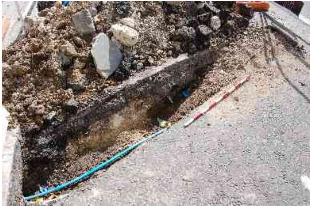
Fig 17: Shallow VMR trenching on Victoria Gardens outside no 55, looking south and showing a large concrete obstruction in the trench.
