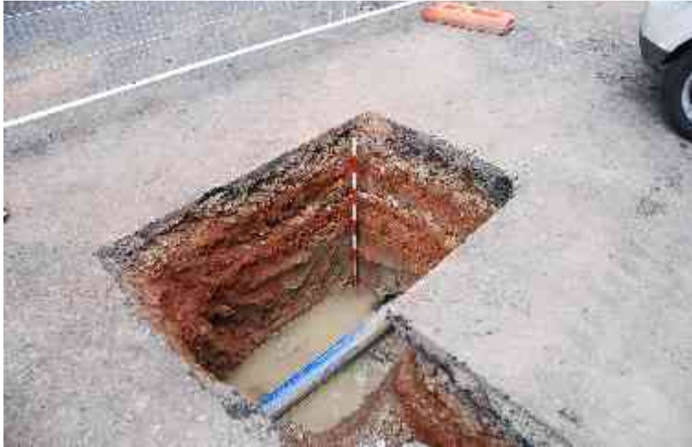
Fig 10: View looking north east of a feeder trench through which the new water main was inserted outside 16 Ladbroke Square ( 1m scale ). The dark red deposits are road make up materials, overlying the truncated surface of the natural clay (which is here at a height of +21.4m OD).
