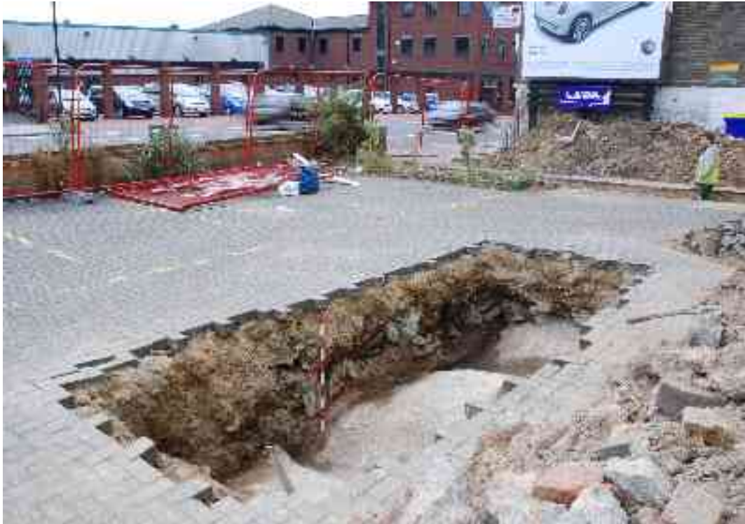
Fig 24 Trench 2: general view looking south towards Tooting High Street
