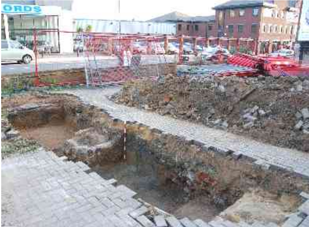
Fig 30 Trench 3: general view looking south towards Tooting High Street
