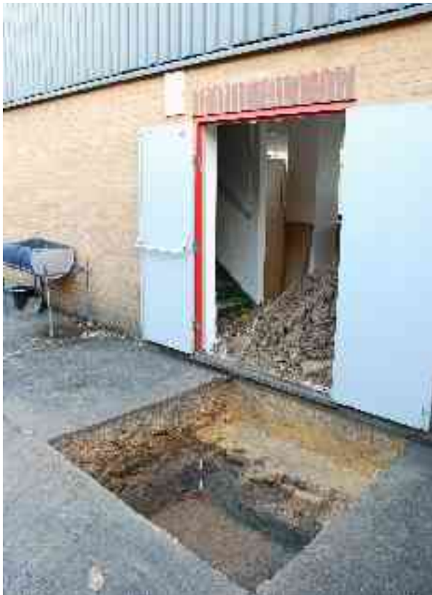
Fig 19 General view of Test Pit 2 looking east
