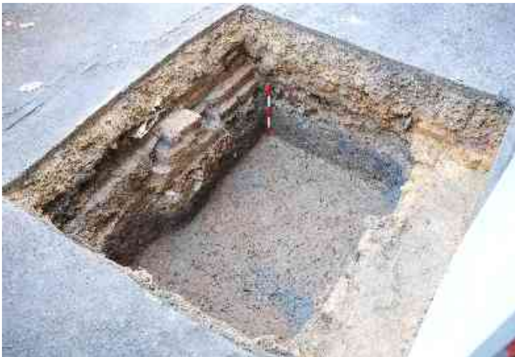
Fig 20 Test pit 2: view looking north, with the brick and concrete wall base [12] to the left ( 0.5m scale )
