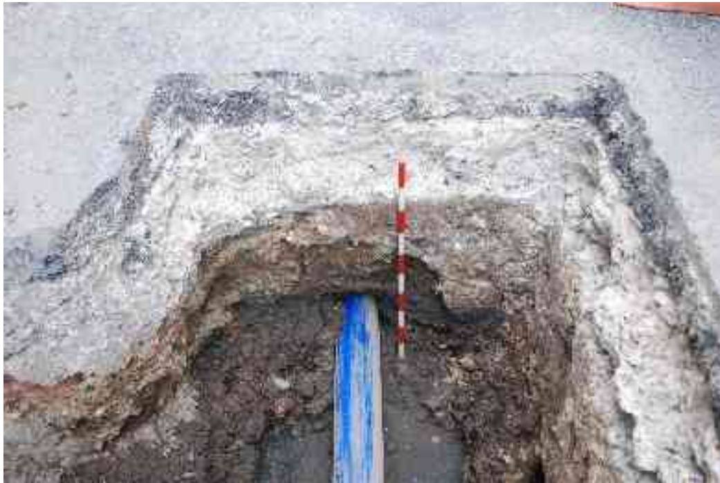
Fig 8 A typical section from the VMR works on Connaught Street, looking east from outside No 21 and revealing the made ground deposits and truncated natural brickearth below the tarmac and concrete hardcore road make up ( 1m scale )
