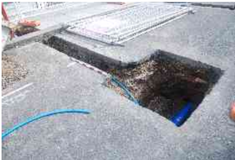
Fig 13 (left) A feeder trench that lay adjacent to the east kerb outside No 32 Albion Street. Notice the white chalk layer (modern) that features prominently below the road make up layers
