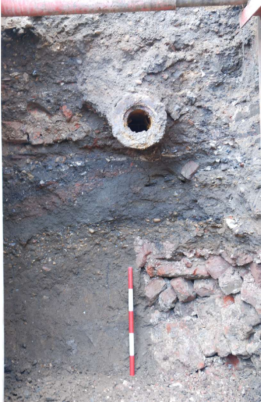
Fig 20 The west (east facing) section of Trench 2 showing the cut (to right of the scale) through the demolition layers for the construction trench for the watermain.
