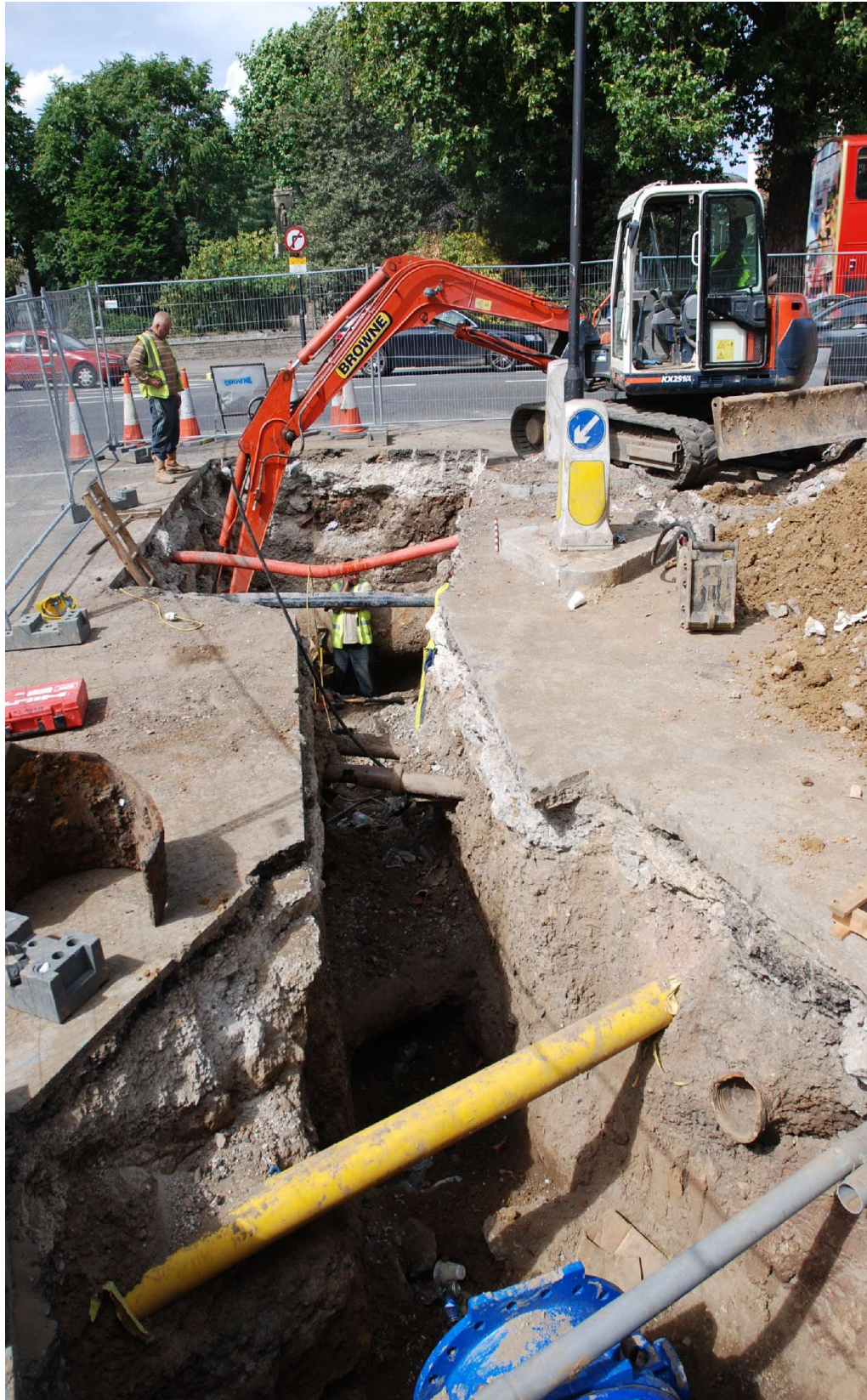
Fig 24 General view of Trench 3, looking northeast.
