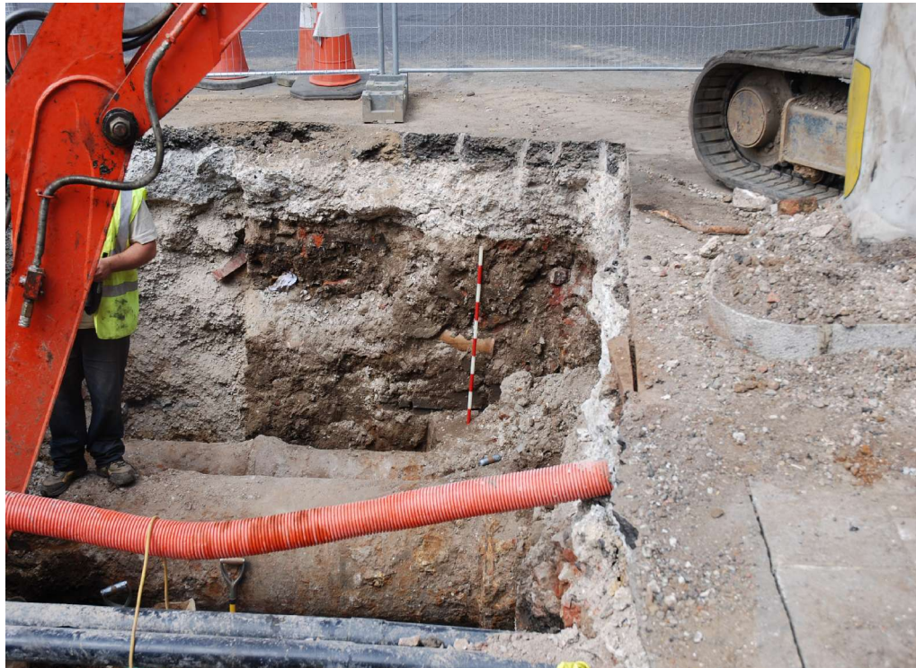
Fig 25 Distinct strata in Trench 3, cut by large block of modern concrete to the west, these deposits are all broadly contiguous in date and relate to the road construction works after circa 1870.
