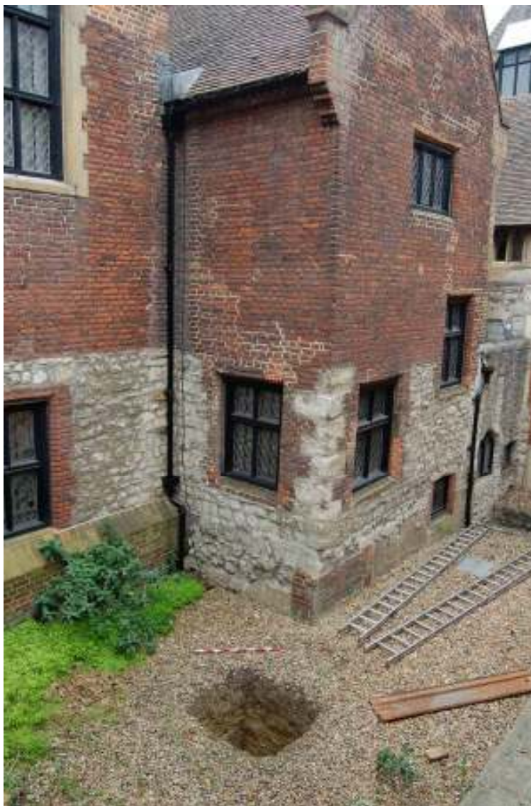
Fig 21 Overhead view showing the location of TP5, looking northwest.
