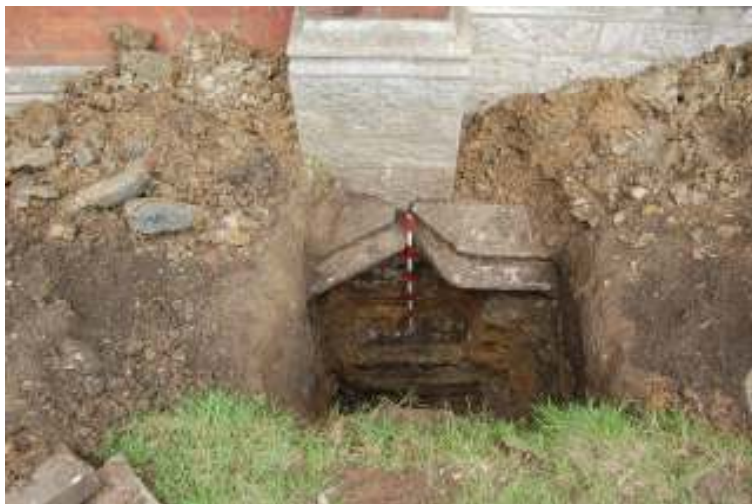
Fig 13 Detail of Test Pit 2 looking down from the raised flowerbed (approximately north). The service pipes can be seen crossing the TP at depth.
