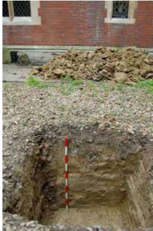
Fig 9 View of TP 5 looking south towards the north wall of the 1890 Lower Bentlif Gallery (where it extends west behind the 1868 gable end of the Queen's Own Royal West Kent Regimental Room). Natural clay can be seen surviving below the gravel covering of the Godiva Courtyard at +14.75m OD.
