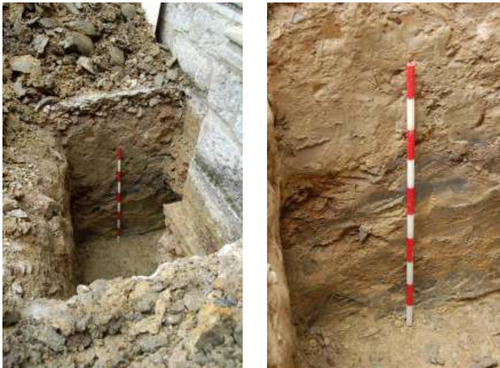
Figure 10 Left: Test Pit 1 looking south, the half brick footer course can be seen in the right side of the image projecting in front of the stone faced pillar. Right: Detail of natural clay geology in TP 1.
