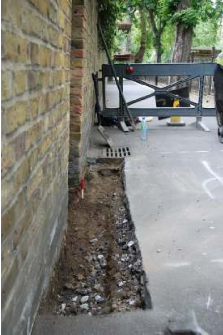
Figure 6 Detail of the southern trench on Churchwell Path. Scale 0.2m.
