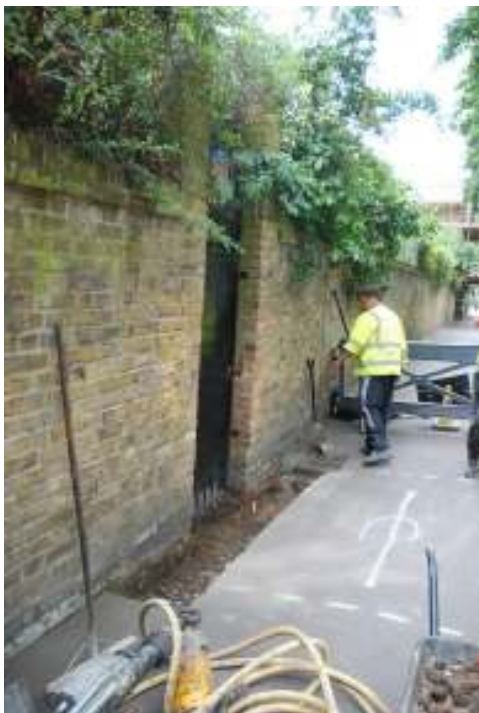
Figure 5 Detail showing the location of the southern trench in front of the access gate to Sutton Square.
