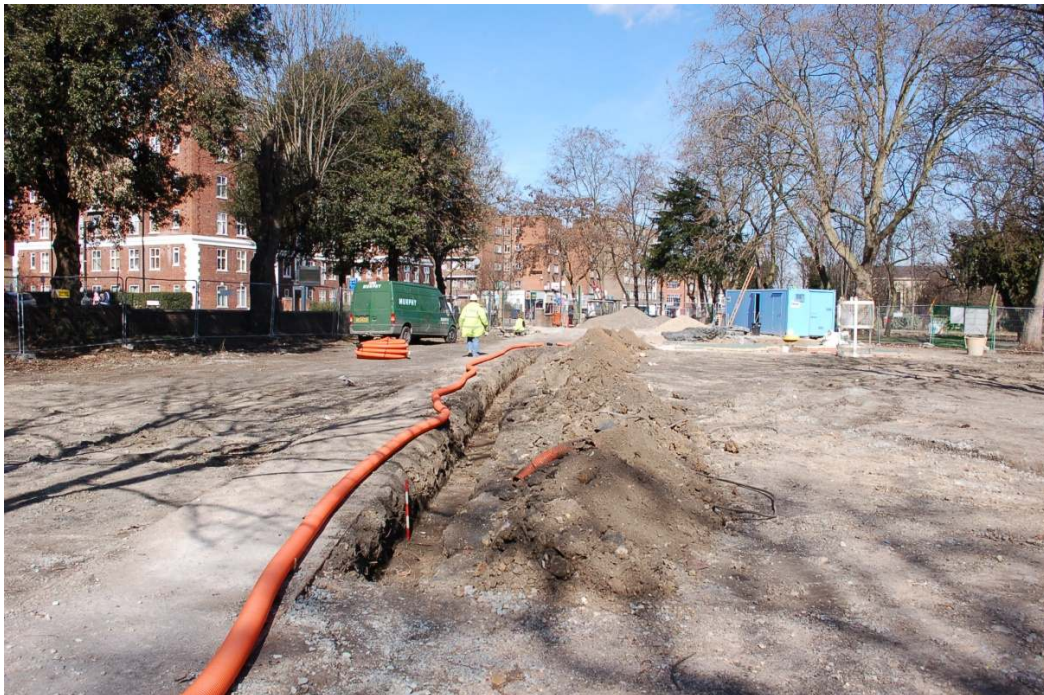
Figure 23: Pipe trenching in Area B (0.5m scale).
