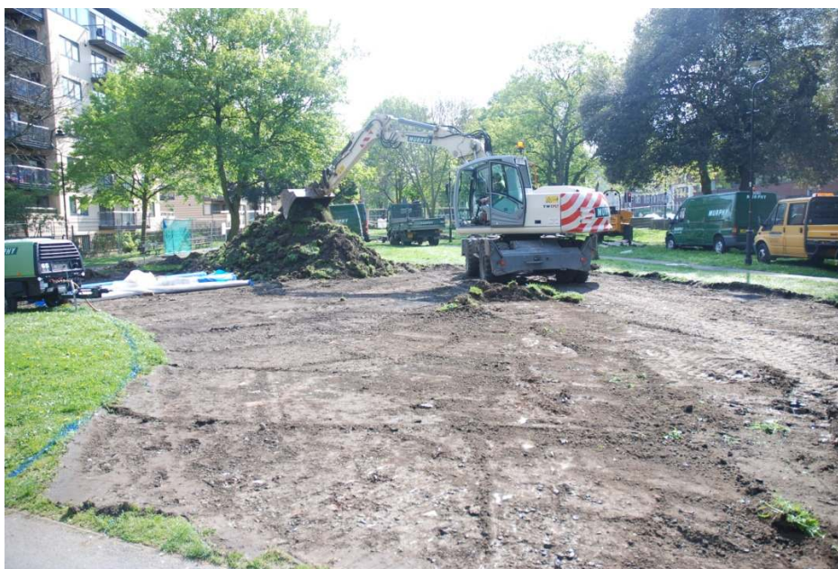
Figure 13: Topsoil stripping in northern half of Area B.
