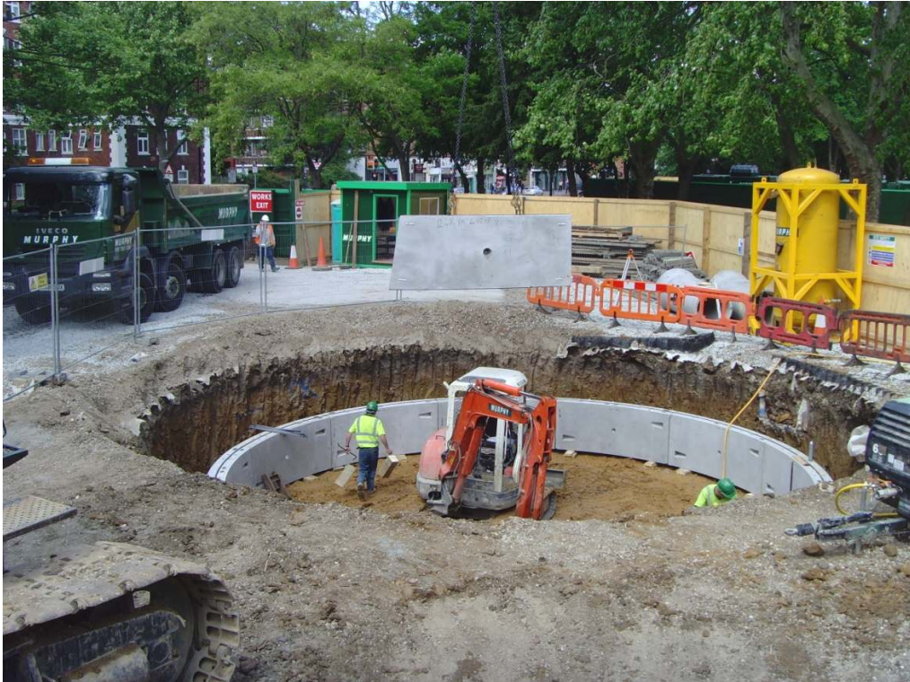
Figure 24: Excavation of the main drive shaft.
