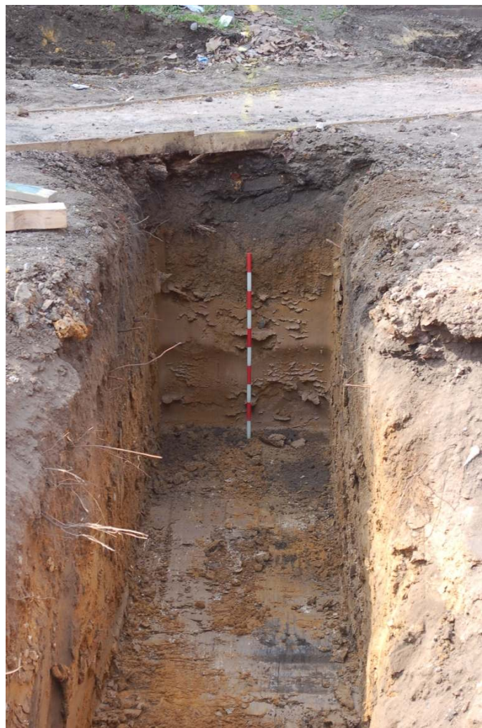
Figure 22: Trenching between the ventilation column and drive shaft (1m scale).
