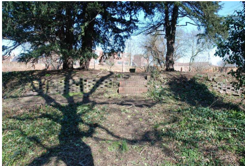
Figure 4: The bastion planted with yew trees and retained by a Honeycomb dry-laid brick wall and red-brick steps.
