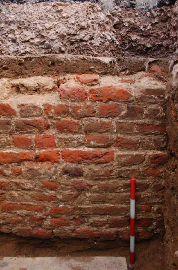
Fig. 7 View of the Southern end of the wall
