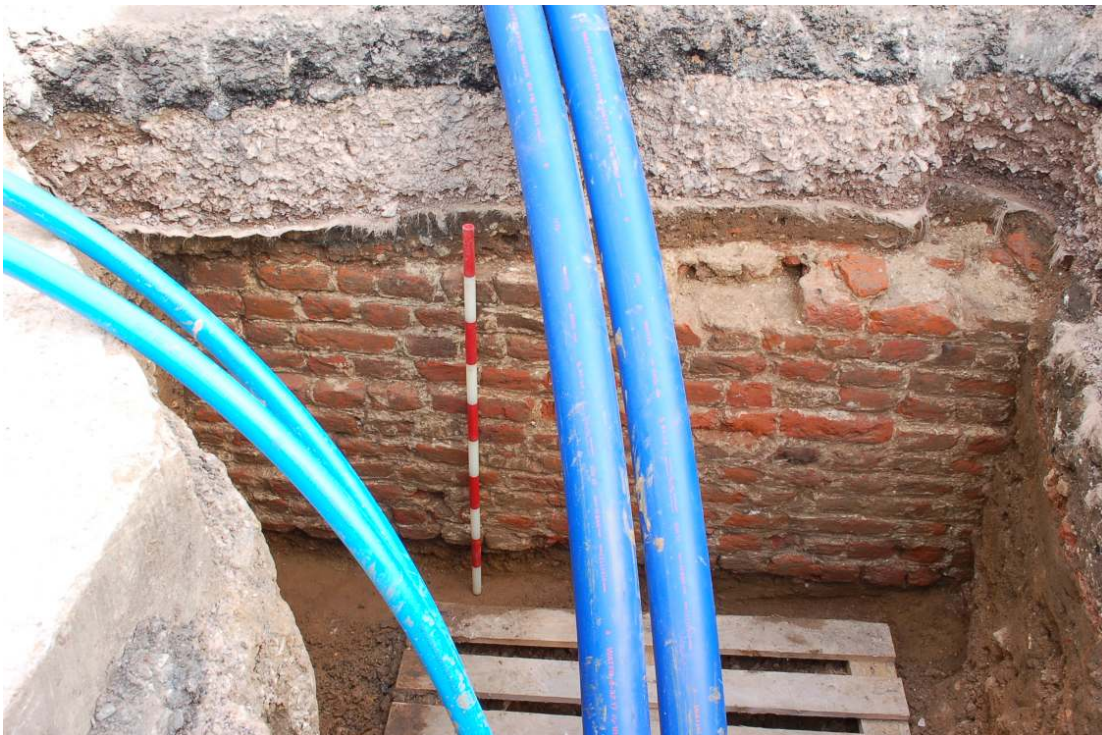
Fig. 6 View of the west face of the wall. Scale 1m.
