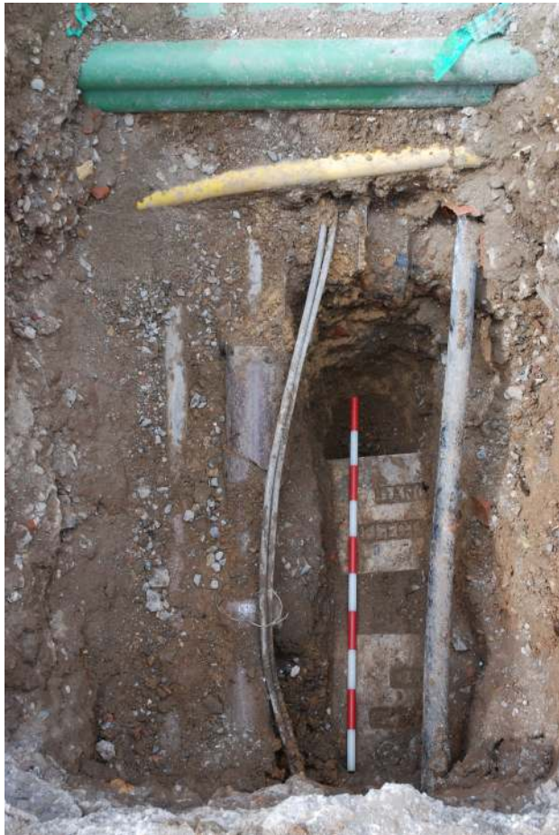
Fig. 7: View of base of pit 4
