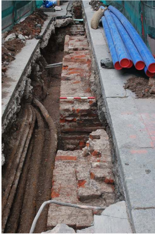
Fig. 16: View along context 6 (brick wall), looking north
