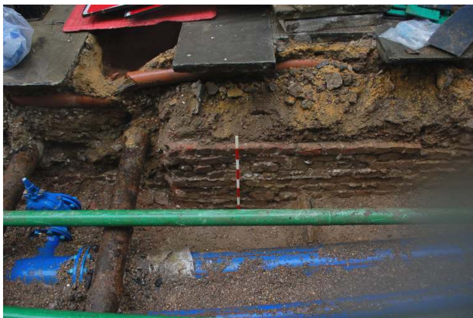
Fig. 34: View of brick wall near the western end of Crosswall
