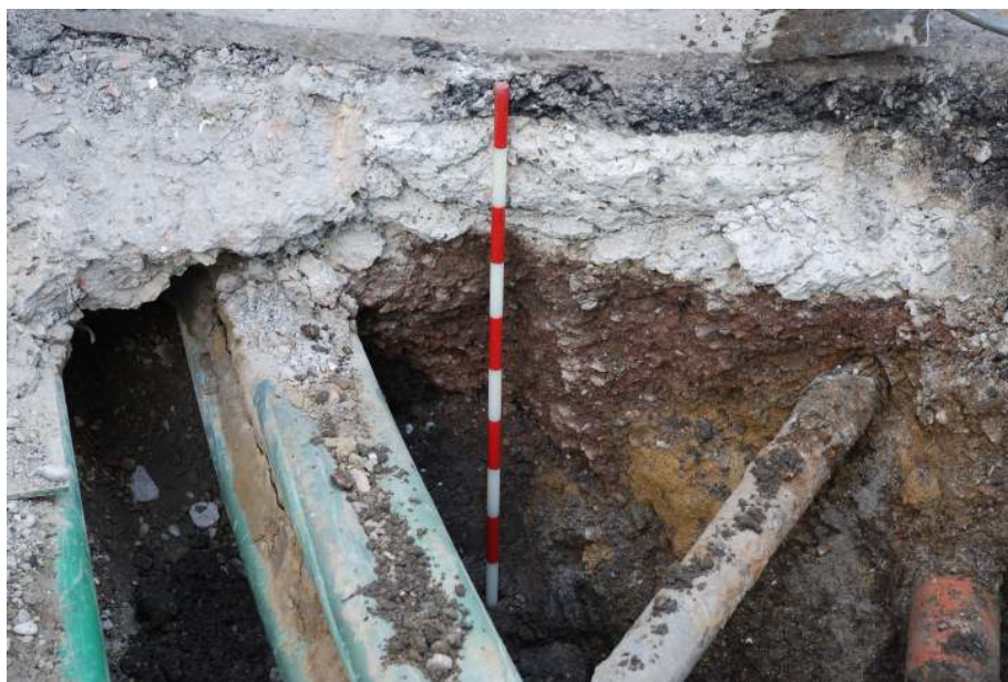
Fig. 30: View of Fenchurch Street trench with MOT Type 1 crushed stone
