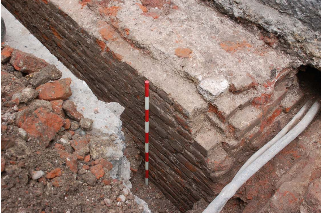
Fig. 18: Close-up view of context 6 (wall)
