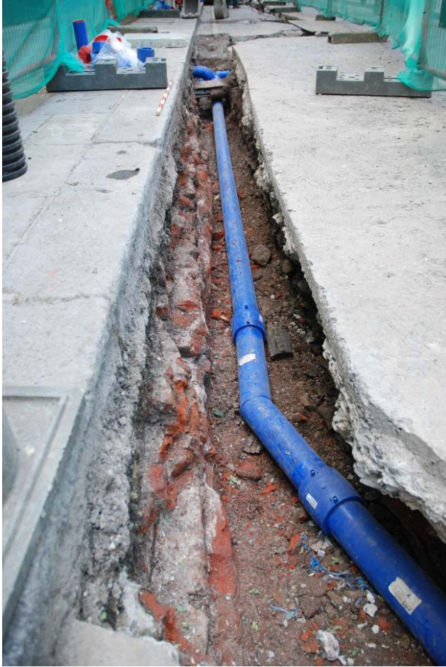
Fig. 26: View along context 13 (brick wall in trench 2), looking south
