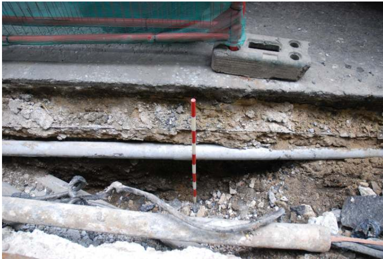
Fig. 25: View of Austin Friars trench (made-ground deposits cut by services under road-surface)
