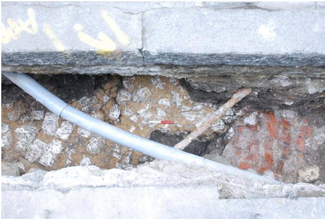
Fig. 16: View of context 10, showing it being truncated by brick-drain (context 14)
