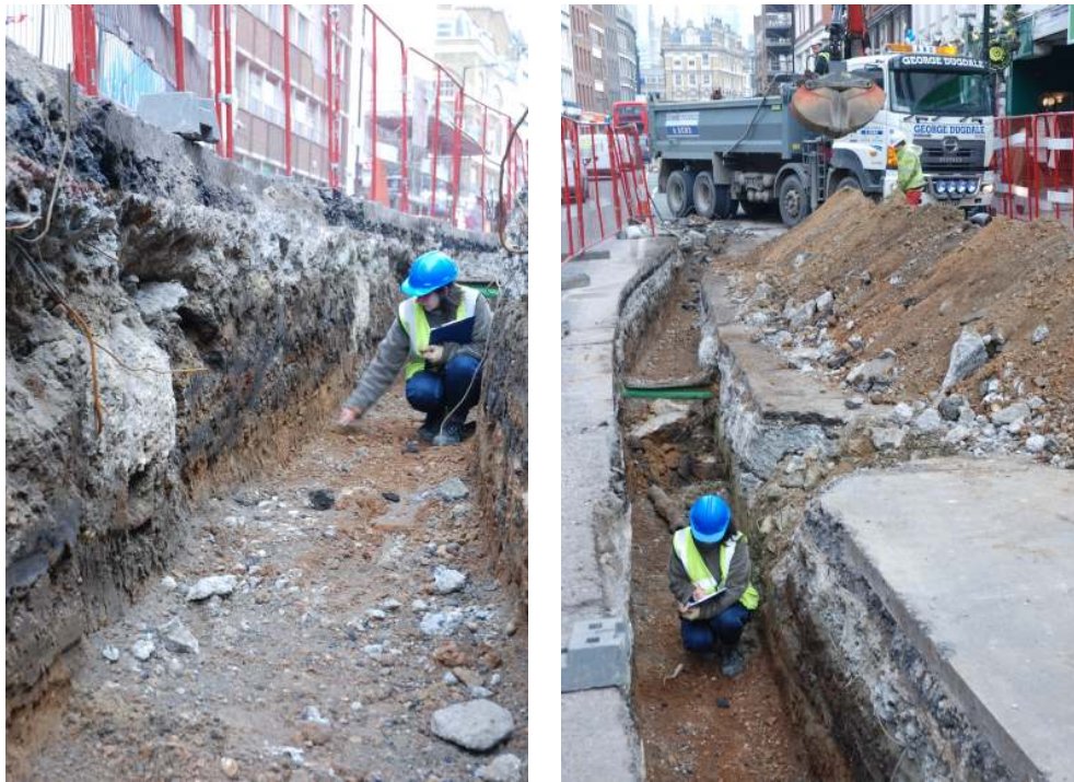
Figure 9: General views in the area of 175 to 191 Borough High Street, outside the Blue Eyed Maid PH and near Chapel Court, showing imported ballast materials, which were encountered in several locations on Borough High Street. This is the historic area of the Marshalsea Prison (to the north) and the King's Bench Prison (to the south), but no archaeological finds or features were present.
