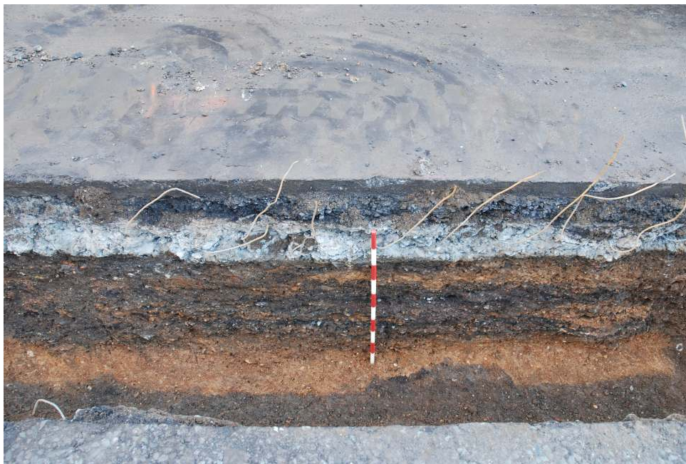
Figure 17: Above: Trenching on the eastern carriageway outside 167 Borough High Street (27/01/10). Below: trench section looking east outside John Harvard Library, 211 Borough High Street showing banded road makeup levels to 1.34m depth. This again is the historic area of the King's Bench and Marshalsea Prisons, but only a residual sherd of grey Roman pottery was recovered and there were no archaeological features.
