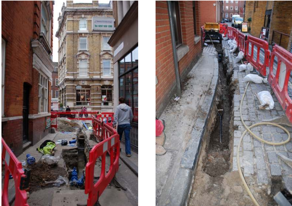
Figure 11: Trenching on Talbot Yard (left) and White Hart Yard (right). Trench works in the yards were generally very shallow and were above the anticipated height of survival of archaeological deposits.
