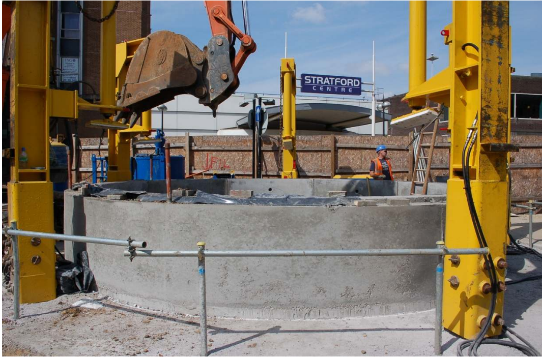
Figure 10: The main shaft outside the Stratford Centre.
