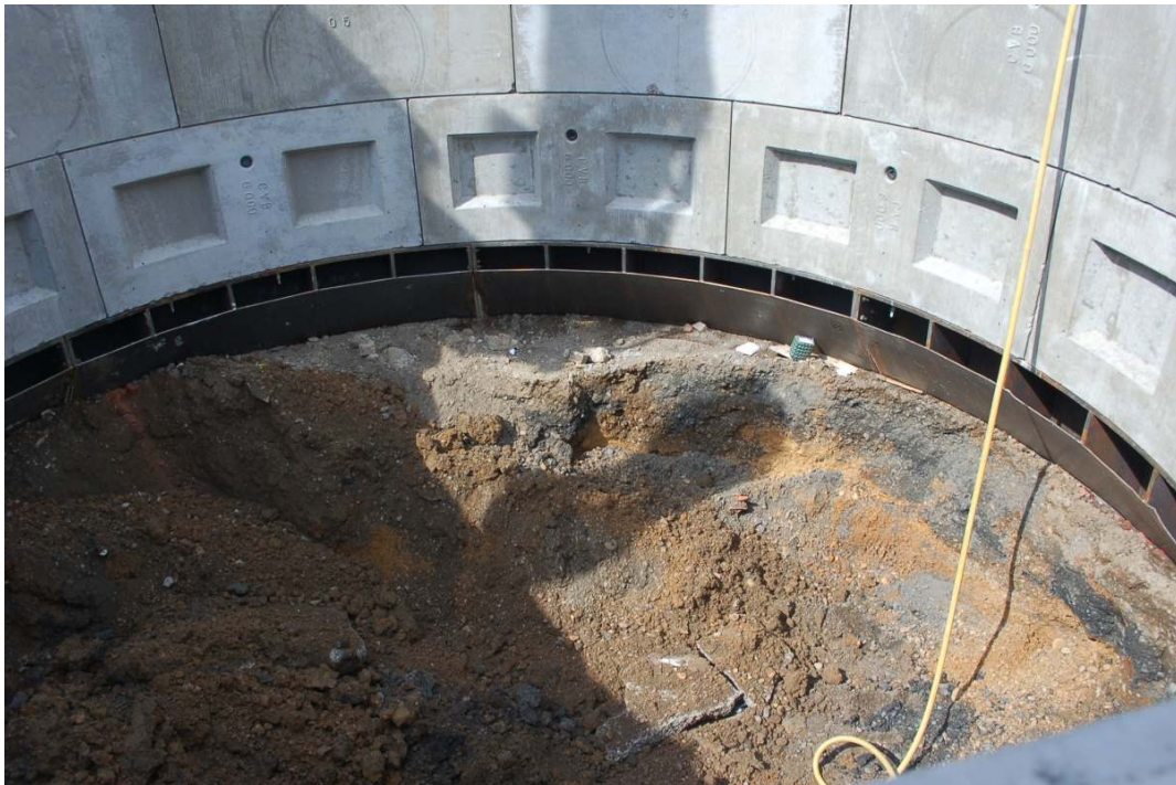
Figure 11: Inside the shaft during excavation showing mixed layers of modern made-ground.
