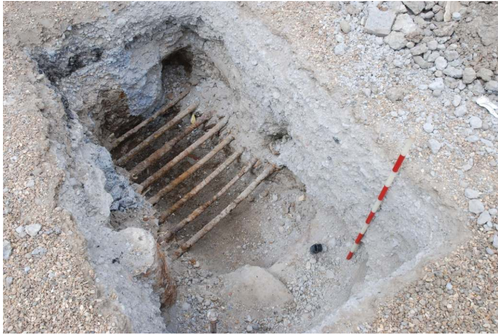
Figure 7: Trial pit A (1m scale).
