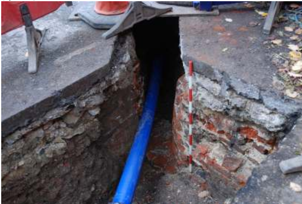
Fig. 60: Photo of brickwork in eastern section and north-eastern corner, trench 49, Bermondsey Wall East
