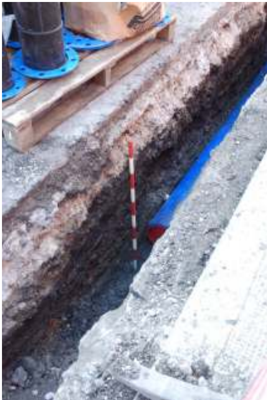
Fig. 38: Photo of trench 27, Paradise Street
