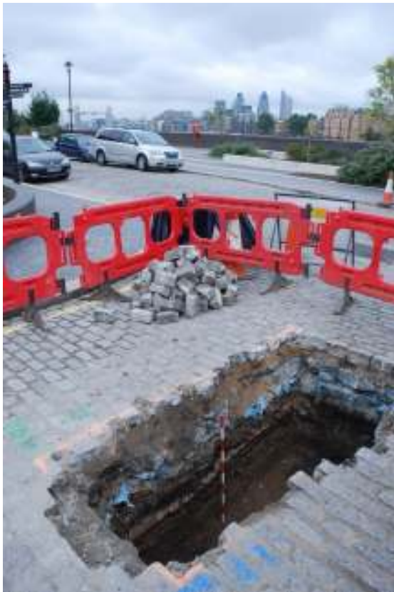
Fig. 49: Photo of trench 38, Cathay Street
