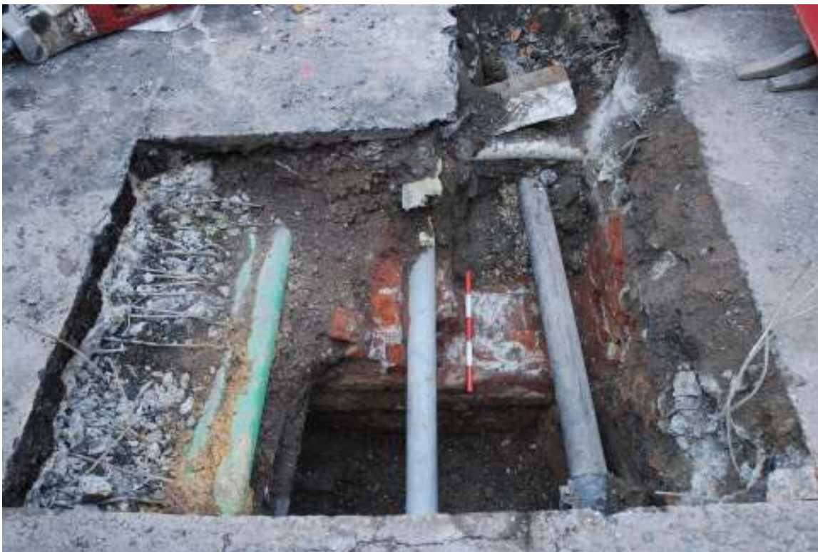
Fig. 44: Photo of trench 37, Cathay Street
