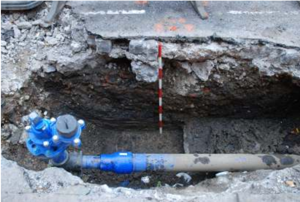
Fig. 14: Photo of trench 19, Cherry Gardens Street
