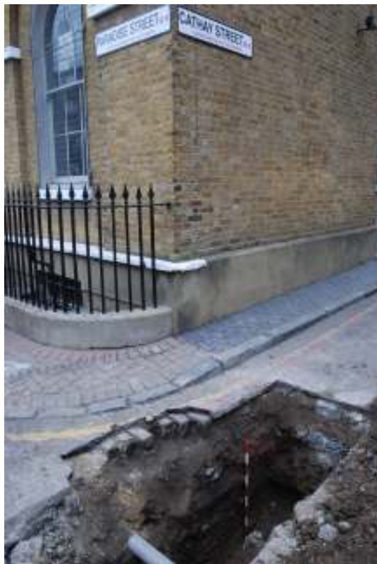
Fig. 42: Photo of trench 39, Cathay Street
