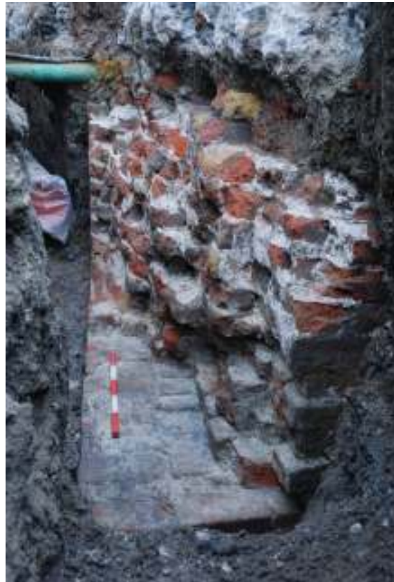
Fig. 23: Photo of Mill Pond Bridge, trench 23, Paradise Street
