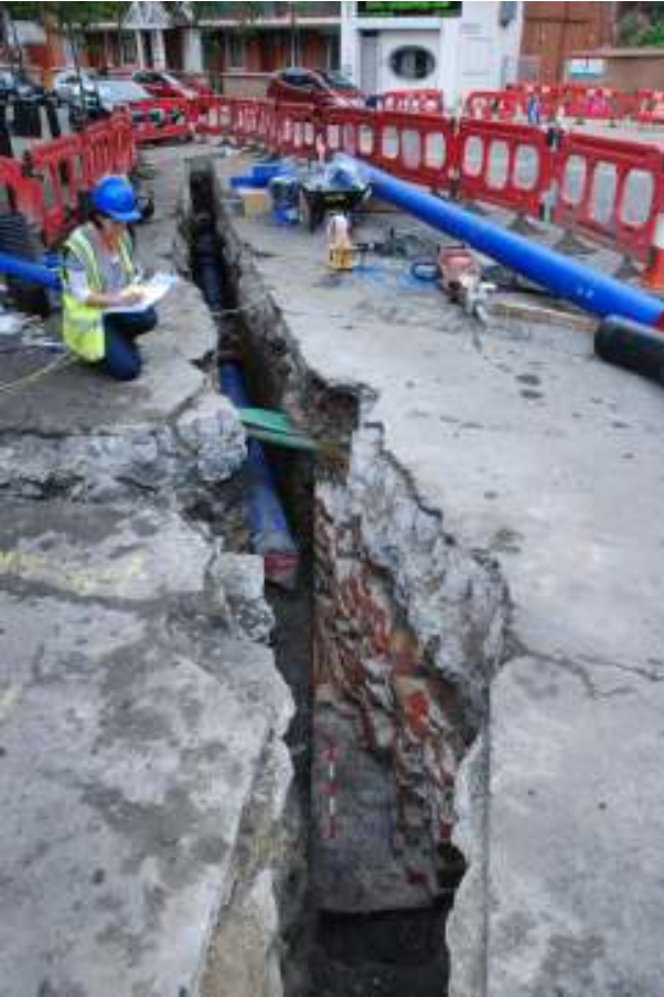
Fig. 22: Photo of Mill Pond Bridge, trench 23, Paradise Street, looking west
