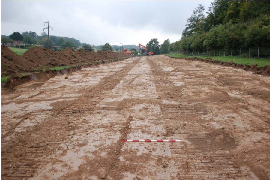
Figure 41: Stripped area for the soakaway excavations, looking southwest towards Cradles Road.
