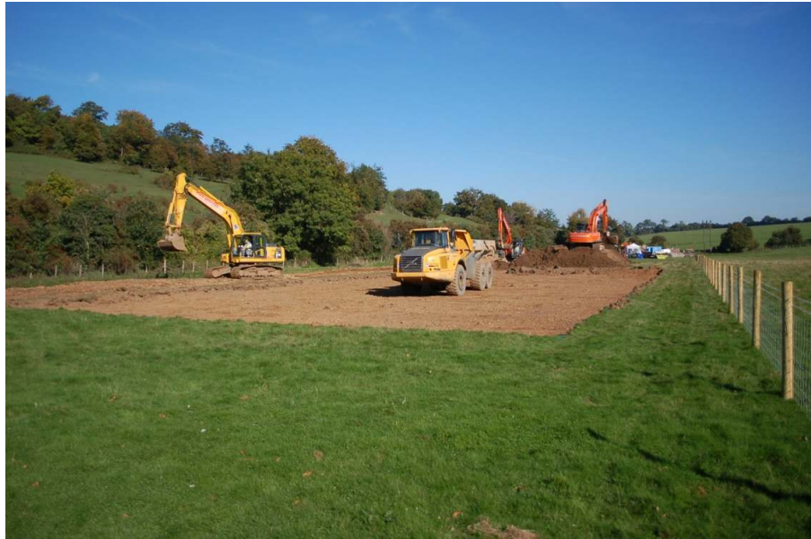
Figure 36: Topsoil stripping for the chalk bund in Field 6.
