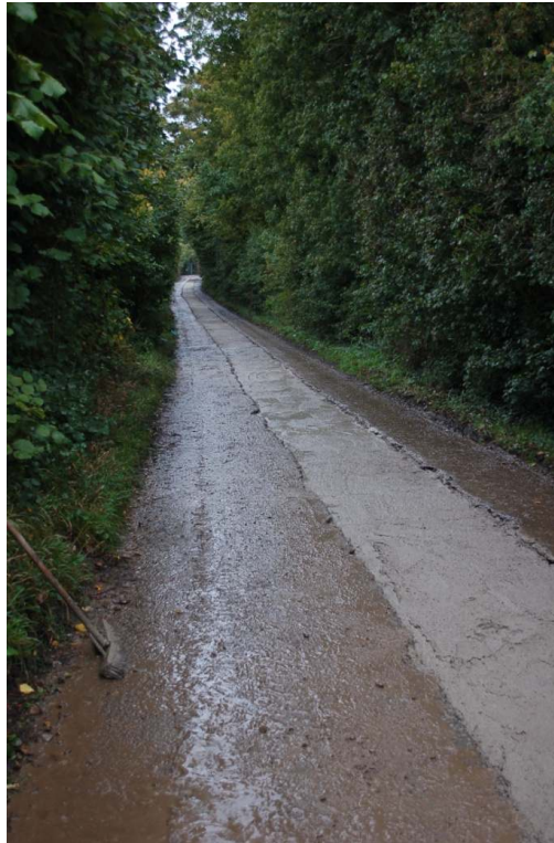
Figure 23: Trenching on Yelsted Road, after backfilling looking north.
