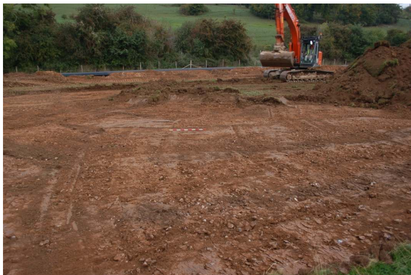
Figure 37: Topsoil stripping for the chalk bund in Field 6.
