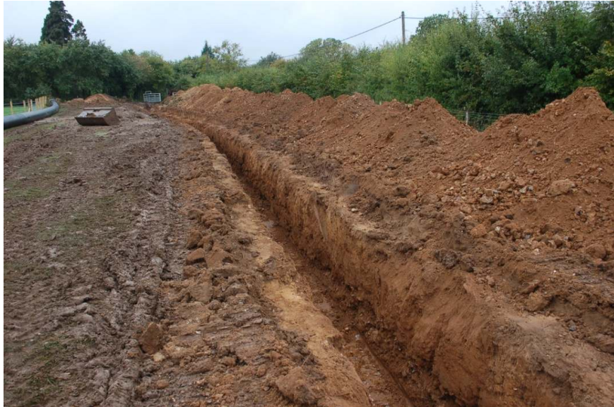
Figure 25: Trenching in Field 4 looking southeast towards the entrance onto Yelsted Road.
