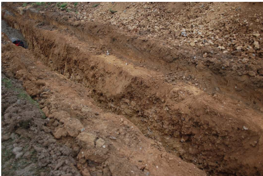
Figure 26: East facing section of pipe trenching in Field 4.
