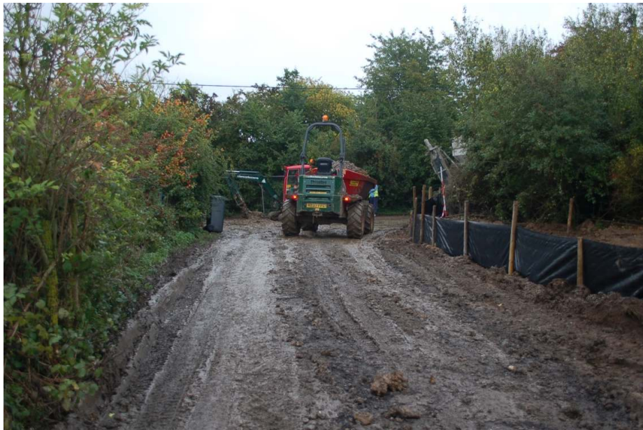
Figure 17: Field 3 at the entrance to Yelsted Road.
