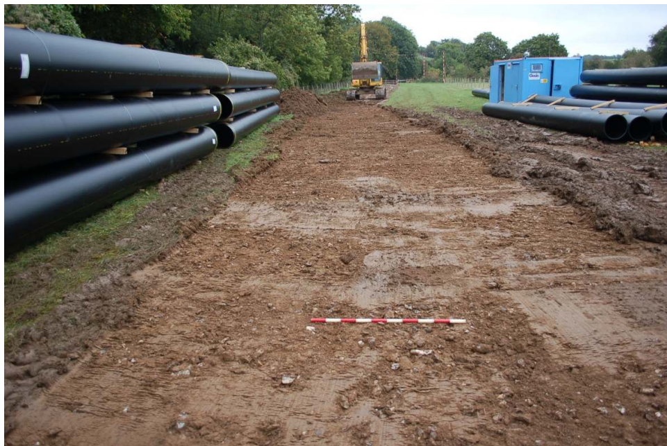
Figure 31: Re-stripping of topsoil, to remove the waterlogged and disturbed overlying deposits (1m scale), looking northeast towards Field 6.
