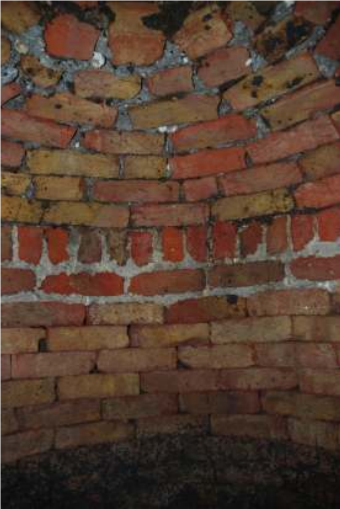
Figure 18: Photo of inside of well [25]
