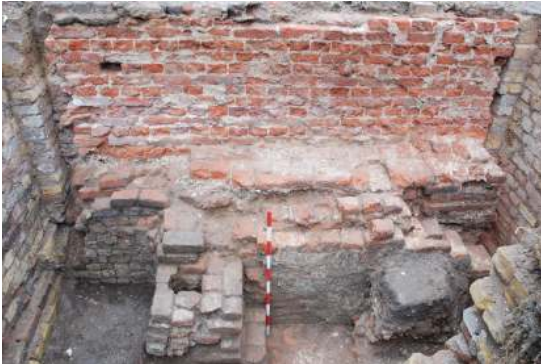
Figure 22: Photo of brickwork [26], to the left of the scale
