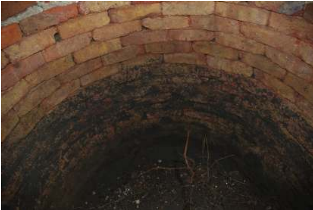
Figure 17: Photo of inside of well [25]
