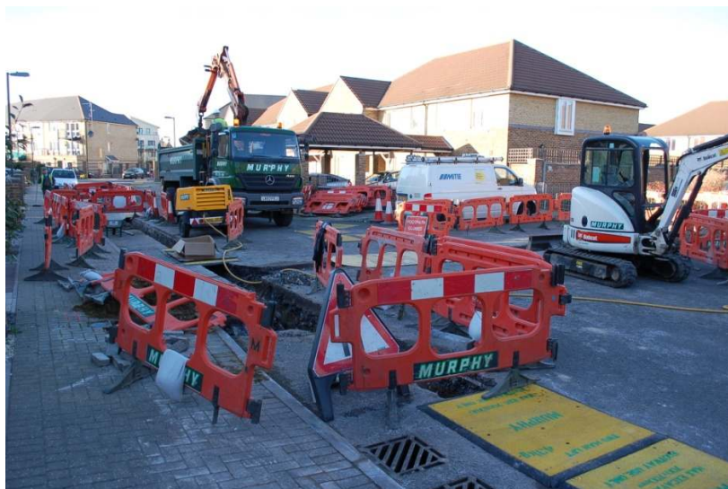
Figure 4: Water mains replacement works on Congo Drive (view south).
