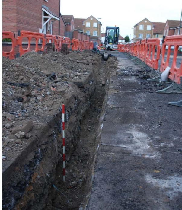
Figure 3: Water mains replacement works on Nile Drive (view west, 1m scale).
