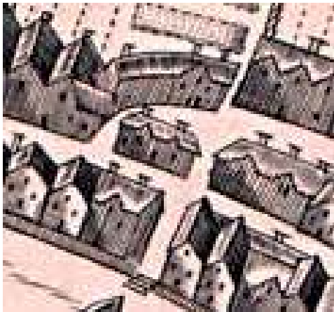
Fig. 55: Newcourt's Map, 1658, clearly showing the roadway and further two houses on the northern side of Narrow Street
