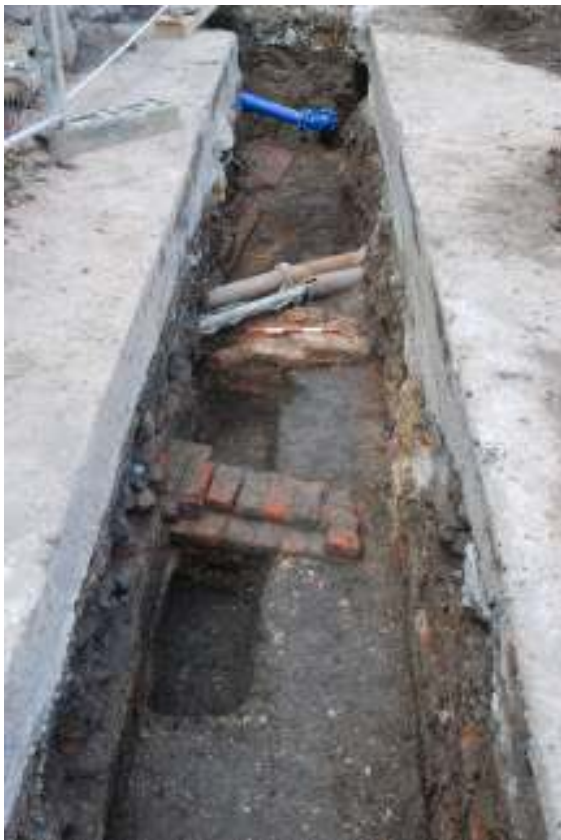
Fig. 57: Photo of brick wall [60], with sondage that revealed the natural river alluvium
