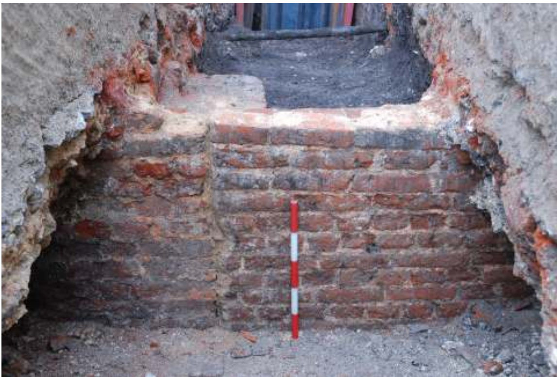
Fig. 39: Photo of the western face of contexts [37]/[38], clearly showing the difference stages of construction of the wall, with the later infill/blocking [37] to the left.
