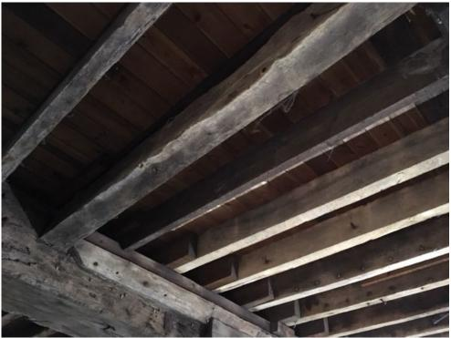
Figure 4: A single common joist sits in its original soffit in bay 3, photograph taken from the south-east (Photograph: Alison Arnold)
