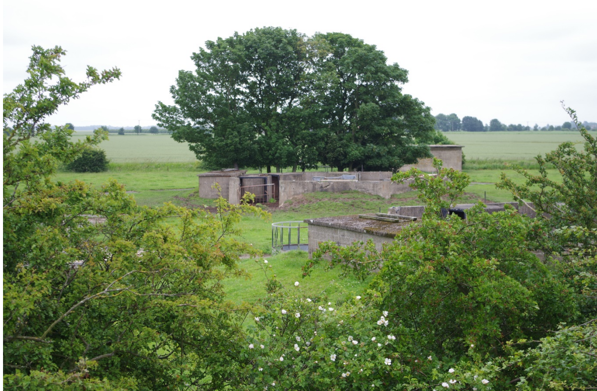
Figure 6.1 Sunk Island Battery – a Scheduled Monument (NHLE 1020187).
