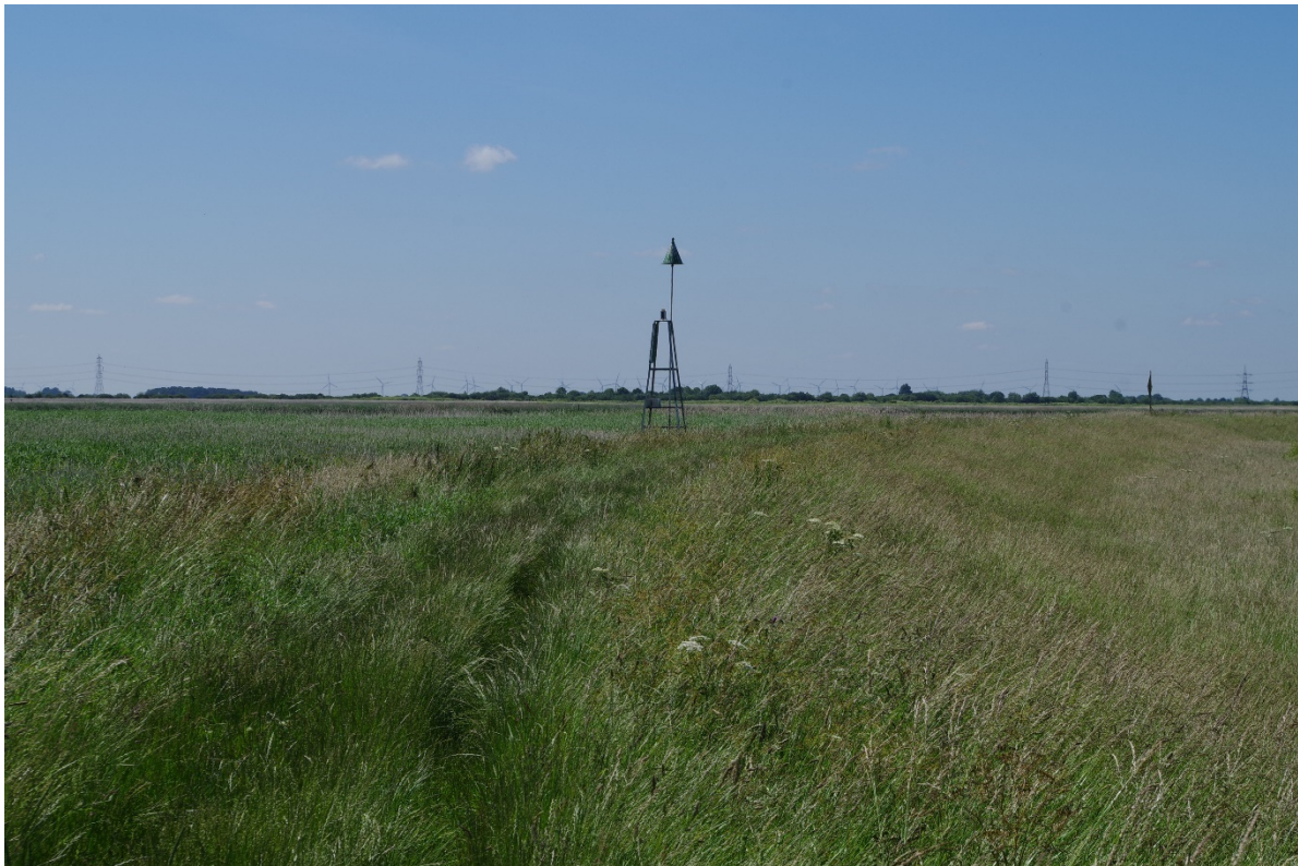
Figure 10.3 A modern navigation beacon built in top of the flood defence bank near Faxfleet, East Riding of Yorkshire.
