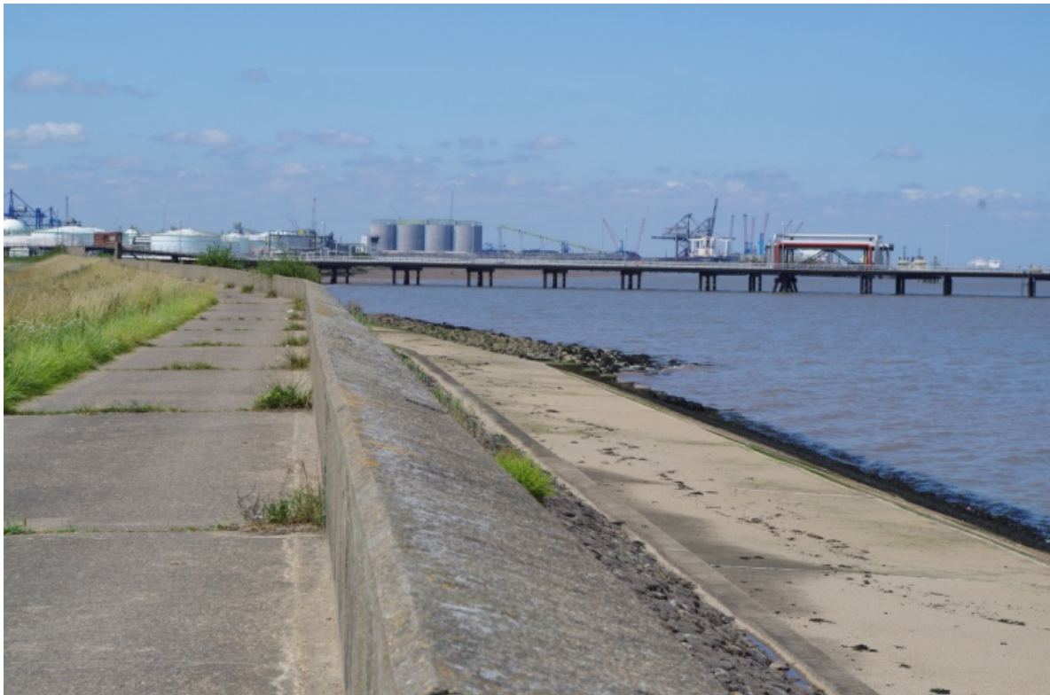
Fig 10.6 Looking to the Port of Immingham from the modern sea defence wall to the north of where Stallingborough Haven was once located. (Photograph taken by CAU in 2015).
